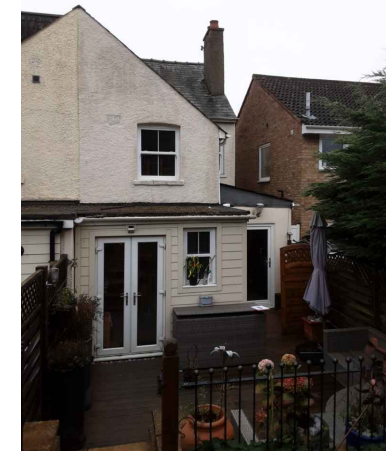
EXISTING PHOTOS - REAR OF PROPERTY
