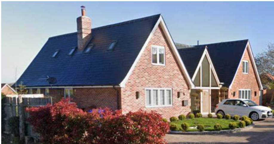
The main, gabled roofs of Willoughby's adopt the same 54 degree pitch
