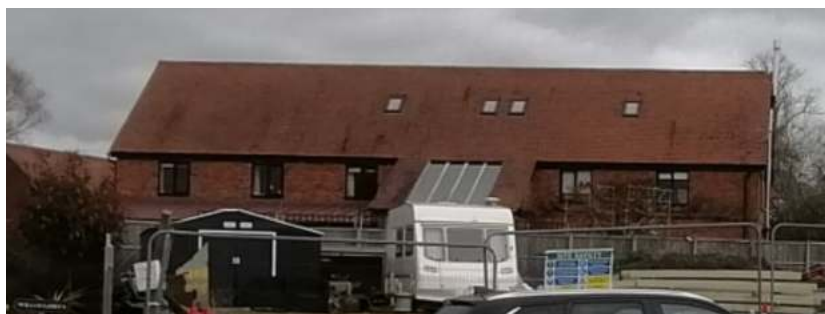
Catslide roof - a traditional feature of the local area, appearing here on Boyton Hall Farmhouse
