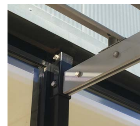
GREY WINDOWS AND FLASHINGS
