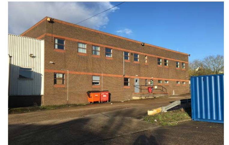
Fig 4- View of Existing Occupied offices
