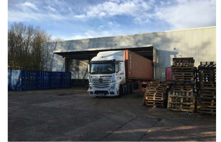
Fig 3- View of Existing Warehouses/Loading docks
