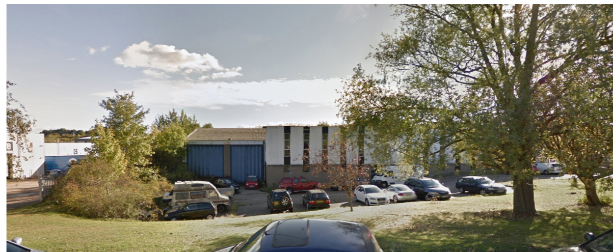
Fig 6 - View of Unit 4 North Elevation
