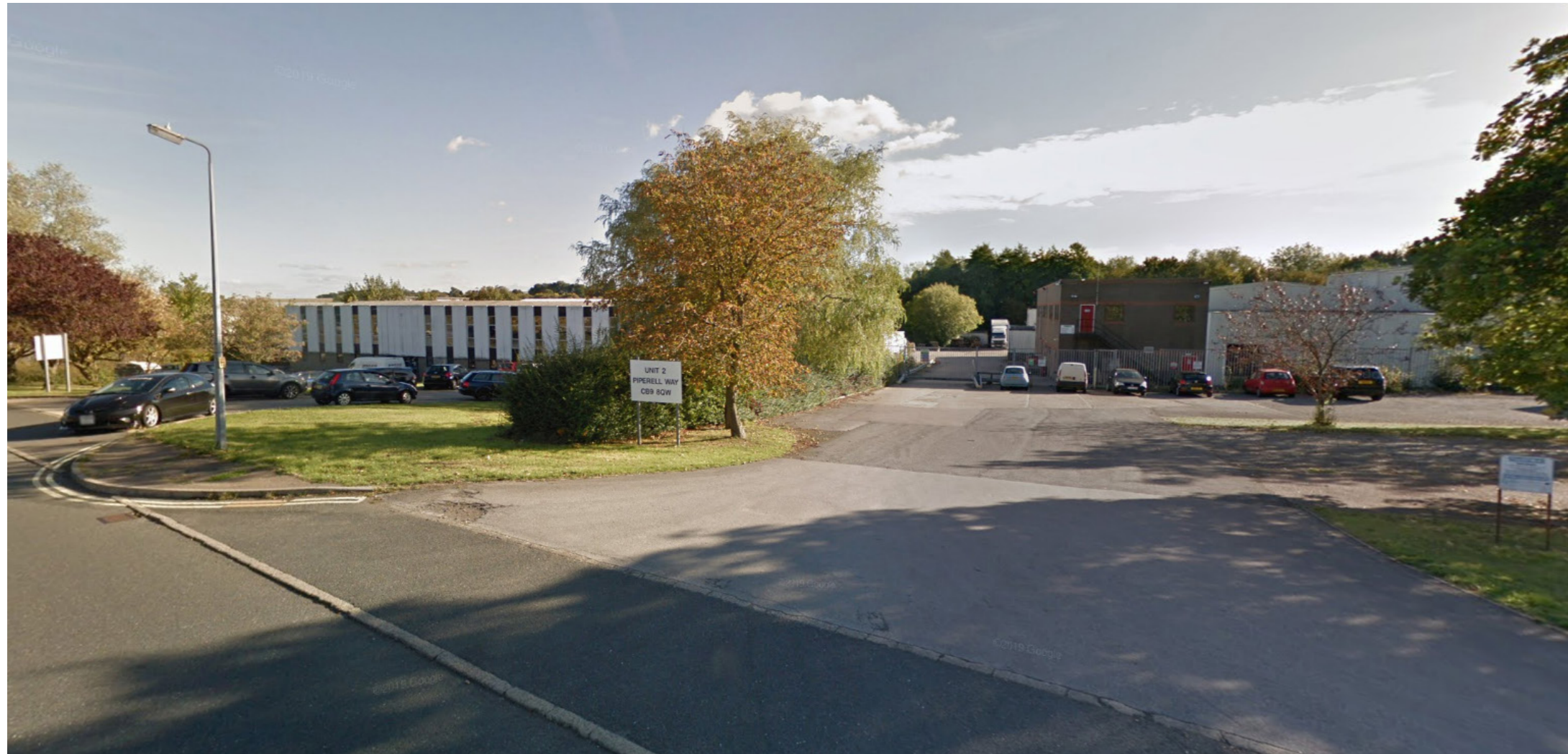
Fig 02 - Site Entrance to Unit 2 Piperell Way
