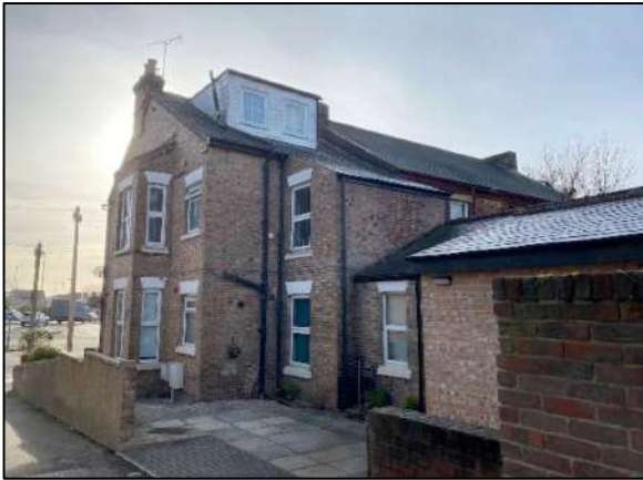
Figure 2: North east flank elevation of No.5 Wrattling Road
