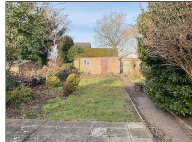
Figure 4: The site, looking north west towards former garage building.
