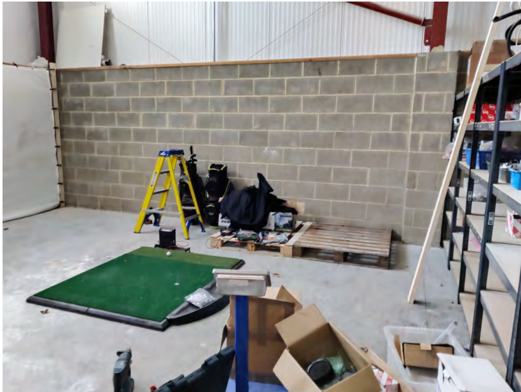
Photo 19: The back of the warehouse building in the eastern building.
