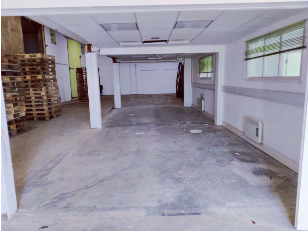
Photo 9: View of the storage area of the western building.
