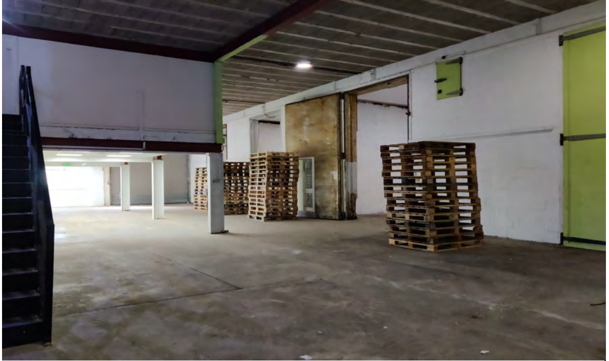
Photo 11: Cold stores, wooden pallets and the stairway up the offices in the western building.
