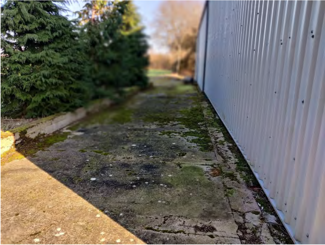
Photo 3: Hardstanding at the north of the Site.
