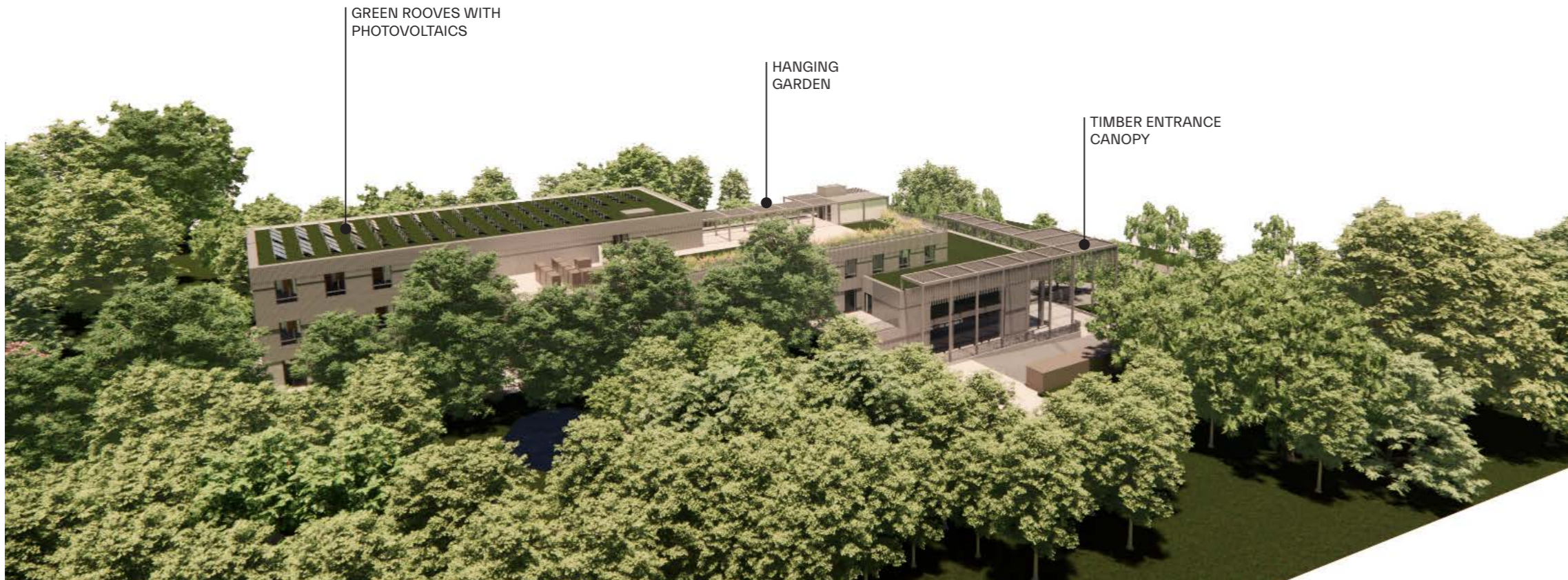
Overhead view from west
