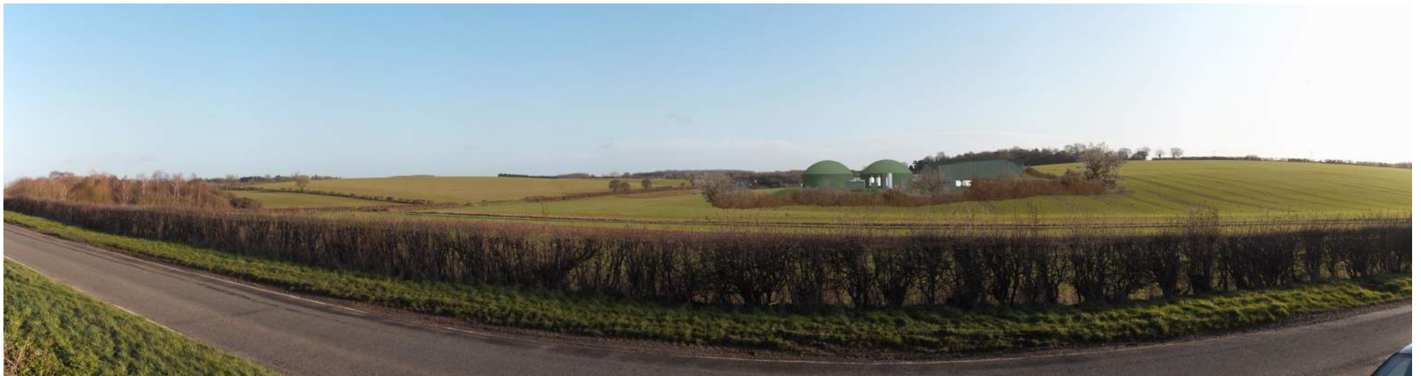
Visualisation of proposed AD Plant Top: prior to landscape mitigation Bottom: with landscape mitigation
