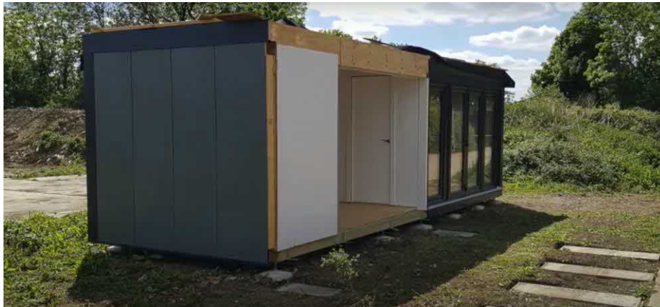
First part in place, note shallow padstones in place in readiness for second part.
