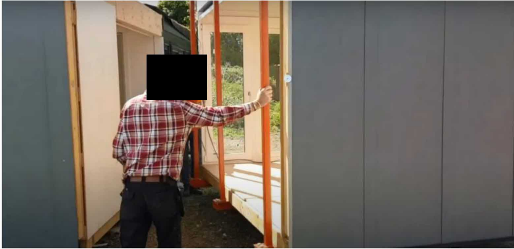
Second half being lifted into place on supporting cradle
