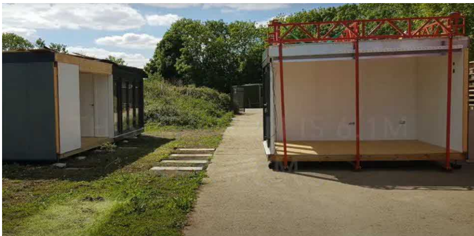
Second part within steel cradle before joining to first part
