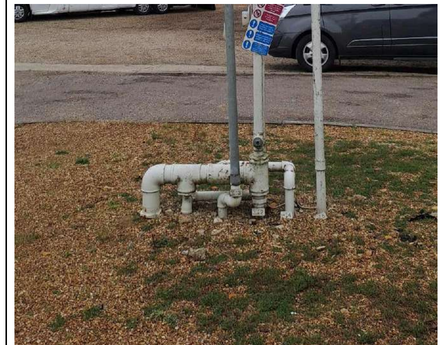
Photo 9: Vents in the centre of the site, to be relocated(16 November 2023)
