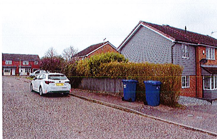
Side Extension at 28 Poplar Close, Haverhil
