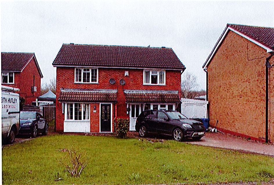
22 Poplar Close (left hand side of the semi detached properties)
