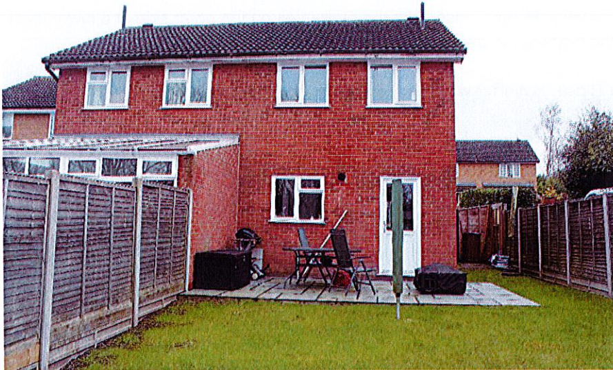
Rear North Elevation of 22 Poplar Close
