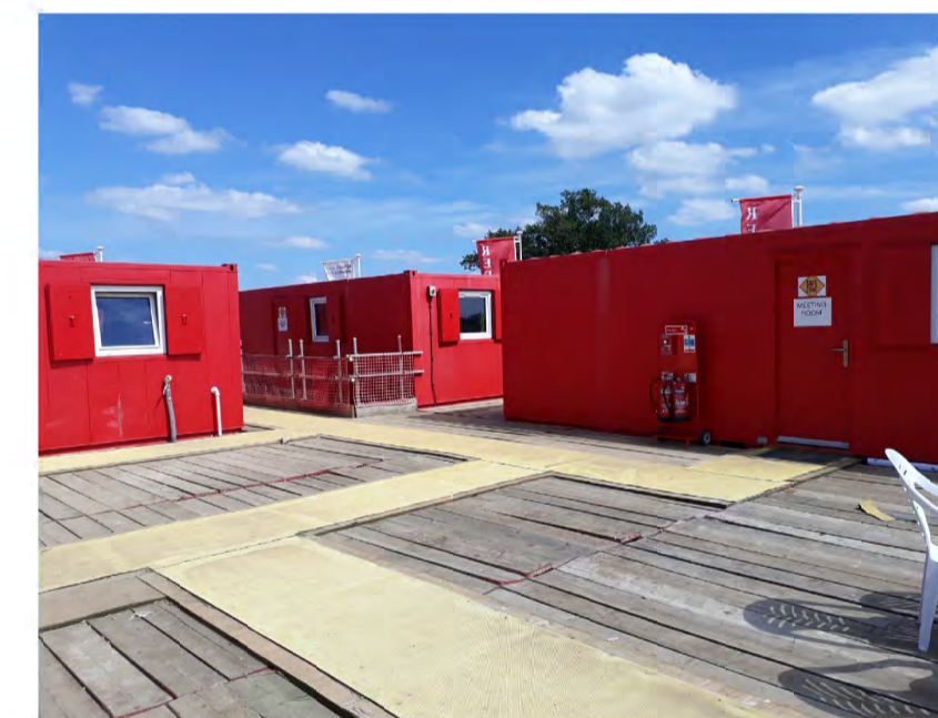
Examples of typical Redrow Compound
