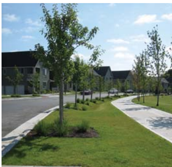
Figure 4c: Swale along road corridor
