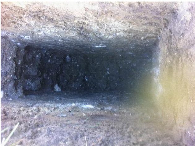
Photo 43: Excavation of trial pit IT22.
