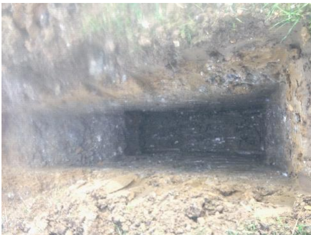
Photo 47: Excavation of trial pit IT24.
