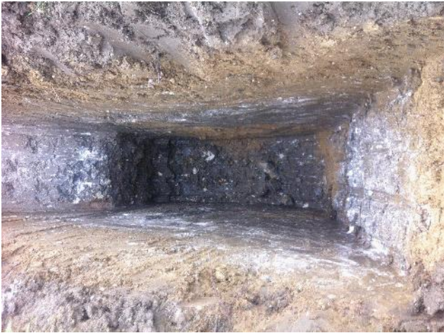
Photo 25: Excavation of trial pit IT13.
