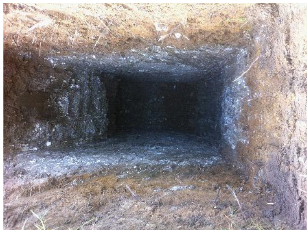
Photo 23: Excavation of trial pit IT12.
