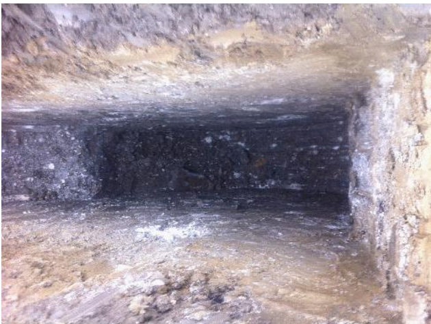
Photo 27: Excavation of trial pit IT14.
