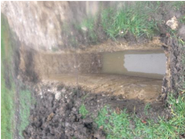
Photo 45: Excavation of trial pit IT23.
