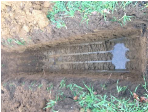
Photo 39: Excavation of trial pit IT20.
