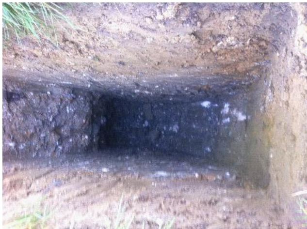
Photo 19: Excavation of trial pit IT10.
