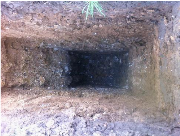
Photo 35: Excavation of trial pit IT18.
