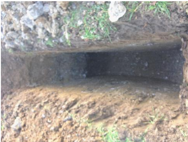
Photo 31: Excavation of trial pit IT16.
