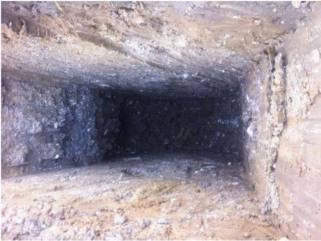
Photo 37: Excavation of trial pit IT19.
