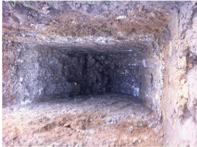
Photo 21: Excavation of trial pit IT11.
