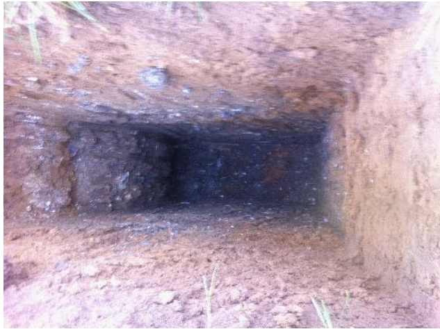
Photo 17: Excavation of trial pit IT09.
