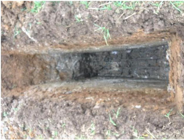
Photo 33: Excavation of trial pit IT17.
