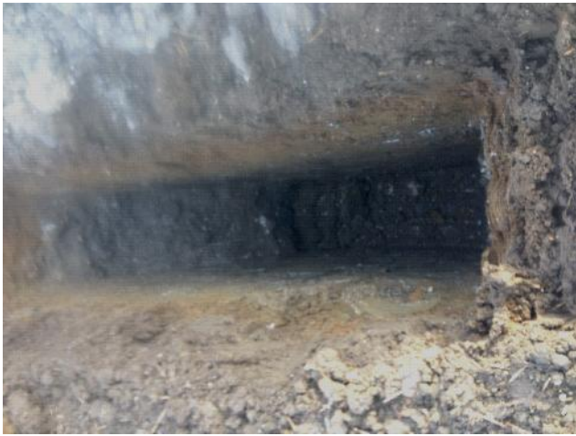
Photo 57: Excavation of trial pit IT25.
