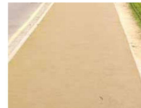
COLOURED CYCLE ASPHALT FOOTPATH/CYCLING
