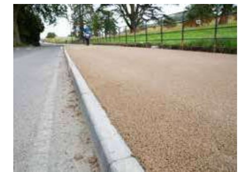
COLOURED ASPHALT PAVEMENT
