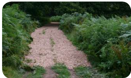
Step 1: Prepare Surface
