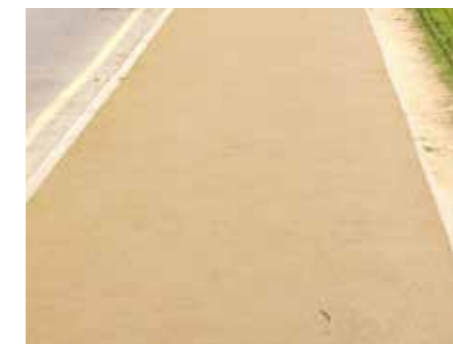
COLOURED CYCLE ASPHALT FOOTPATH/CYCLING
