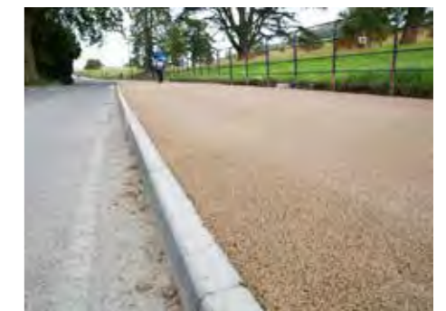
COLOURED ASPHALT PAVEMENT
