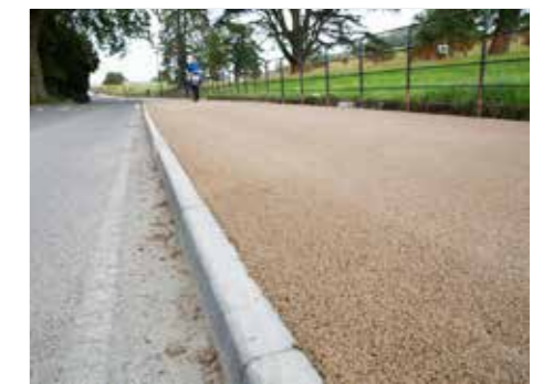
COLOURED ASPHALT PAVEMENT
