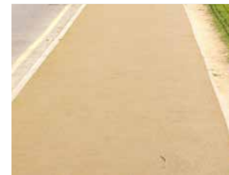
COLOURED CYCLE ASPHALT FOOTPATH/CYCLING
