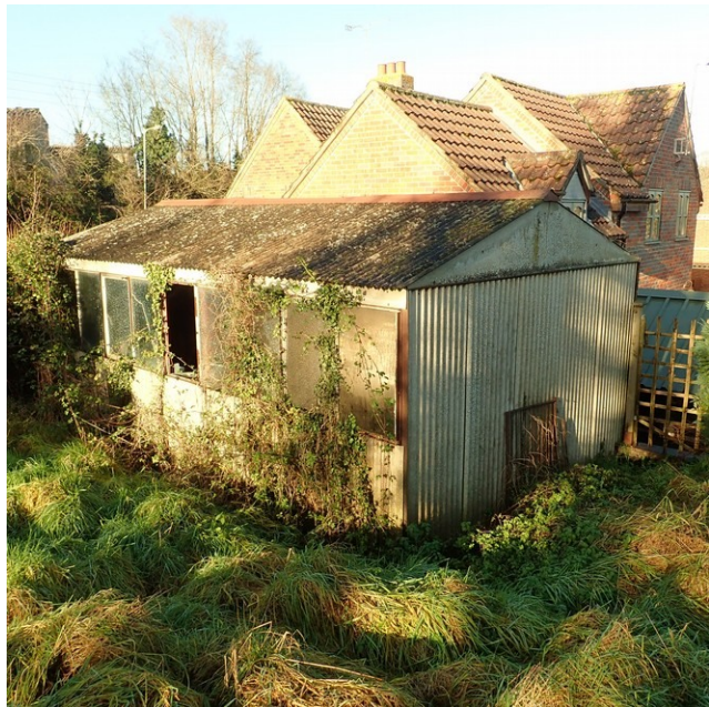
Figure 8: Exterior of garage/workshop
