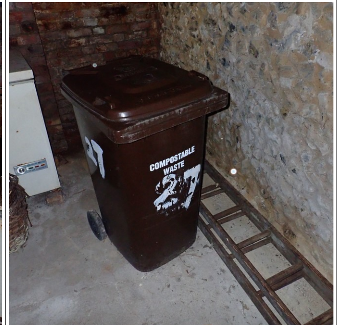
Figure 12: View of south-east corner of undercroft showing well pointed flint wall
