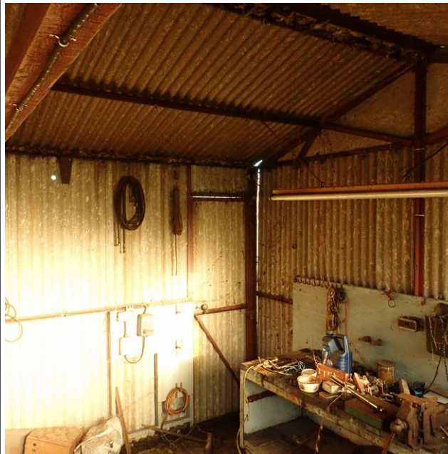
Figure 9: Interior of garage/workshop
