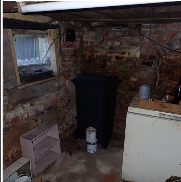
Figure 11: View of North-east corner of undercroft with window
