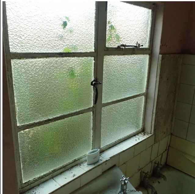
Figure 10: Internal view of bathroom windows, showing thickness of walls
