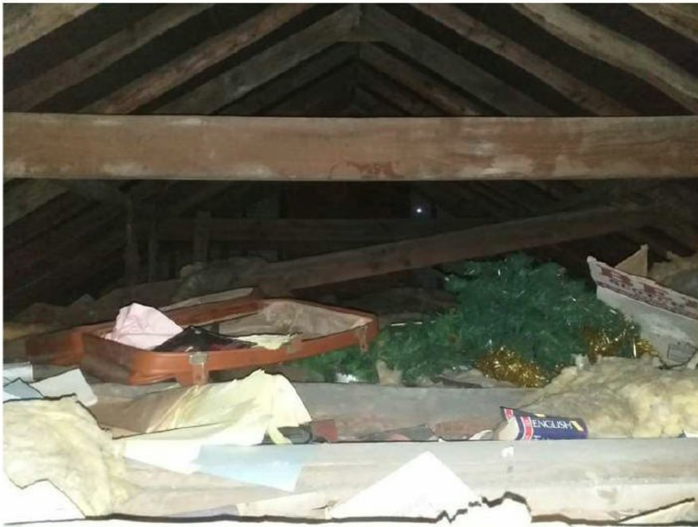
Main building section roof void
