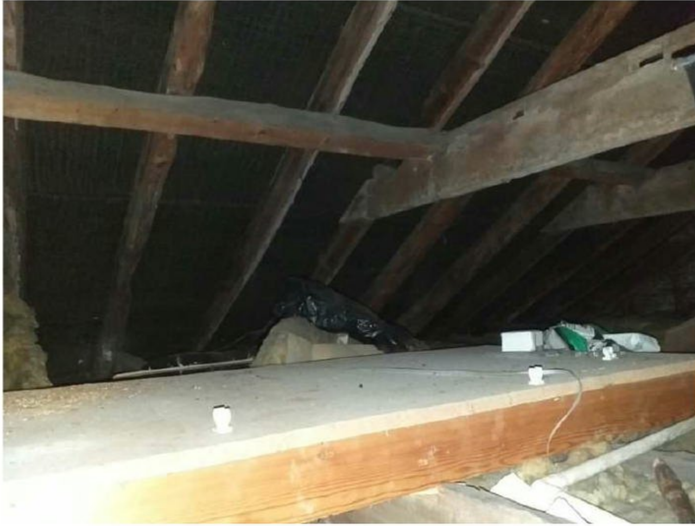
Main building section roof void
