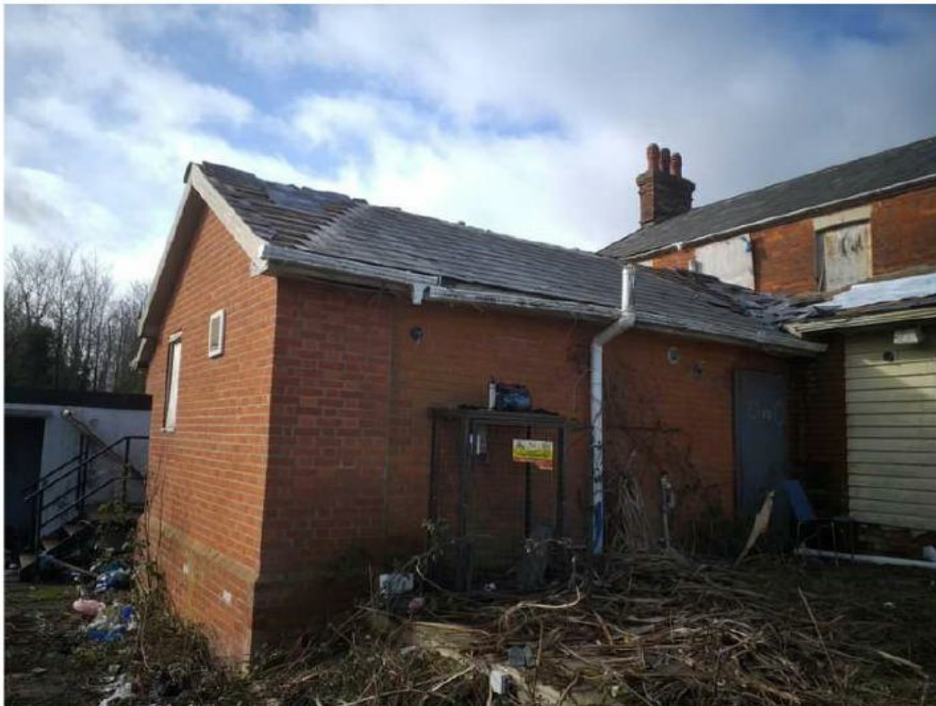
Southern section of building
