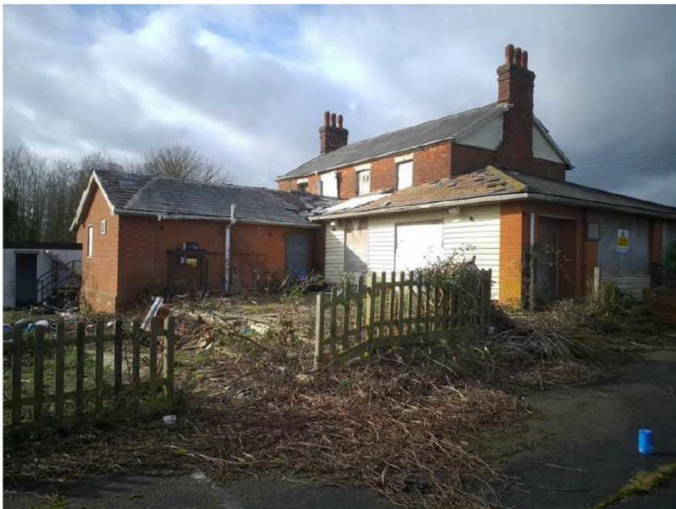
Building viewed from north east
