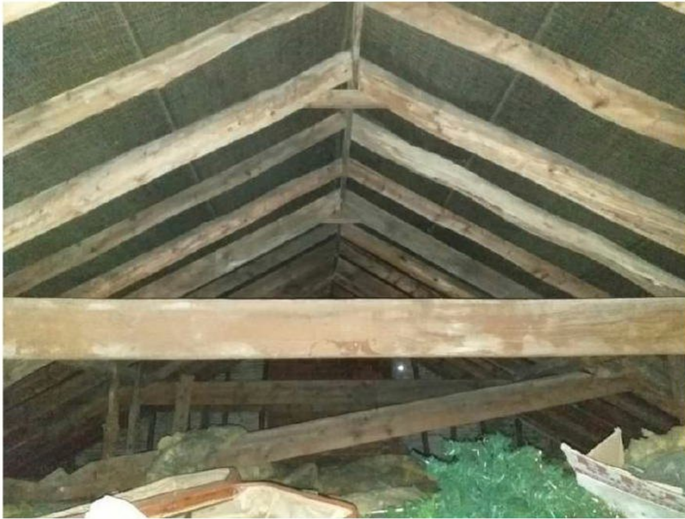
Main building section roof void
