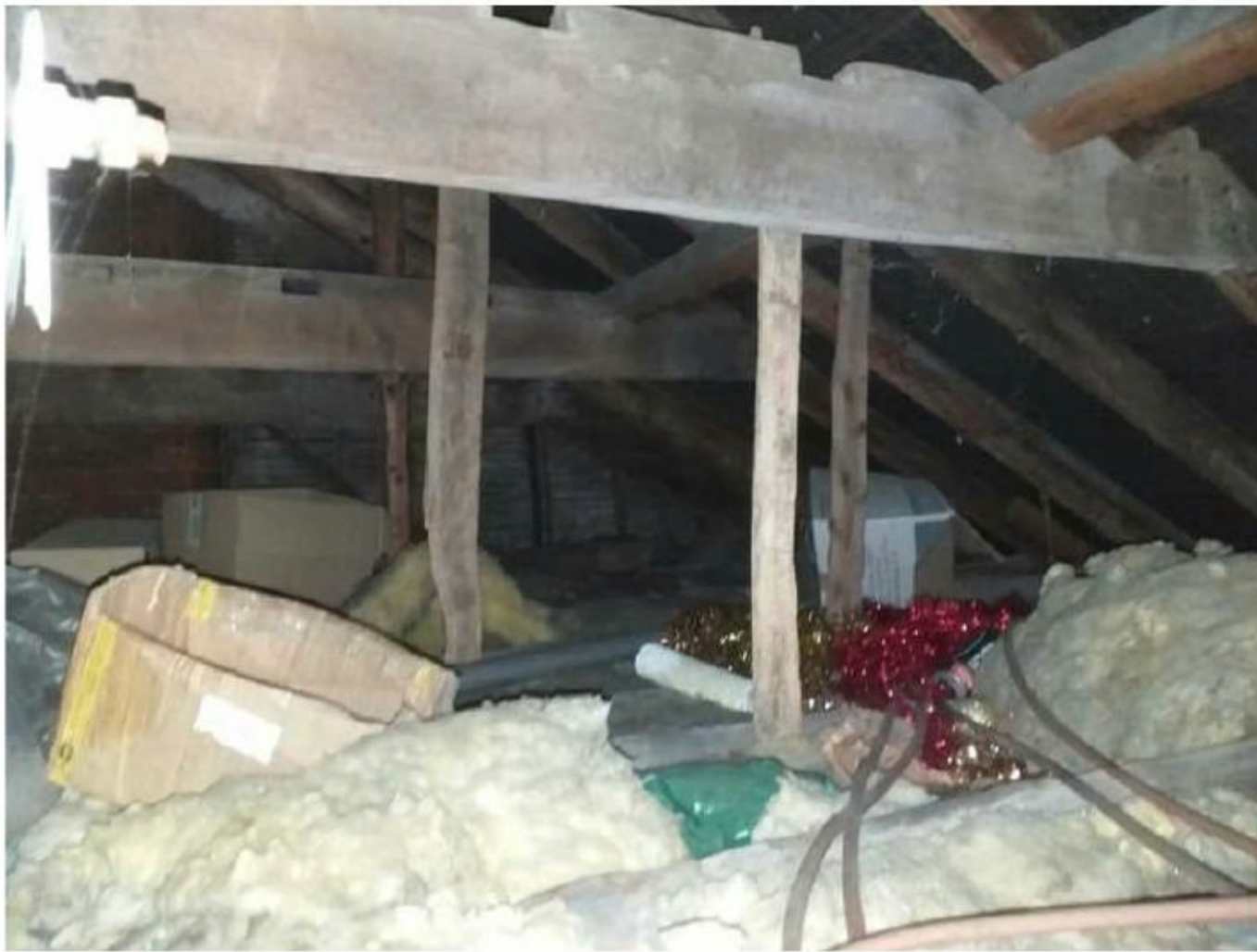
Main building section roof void
