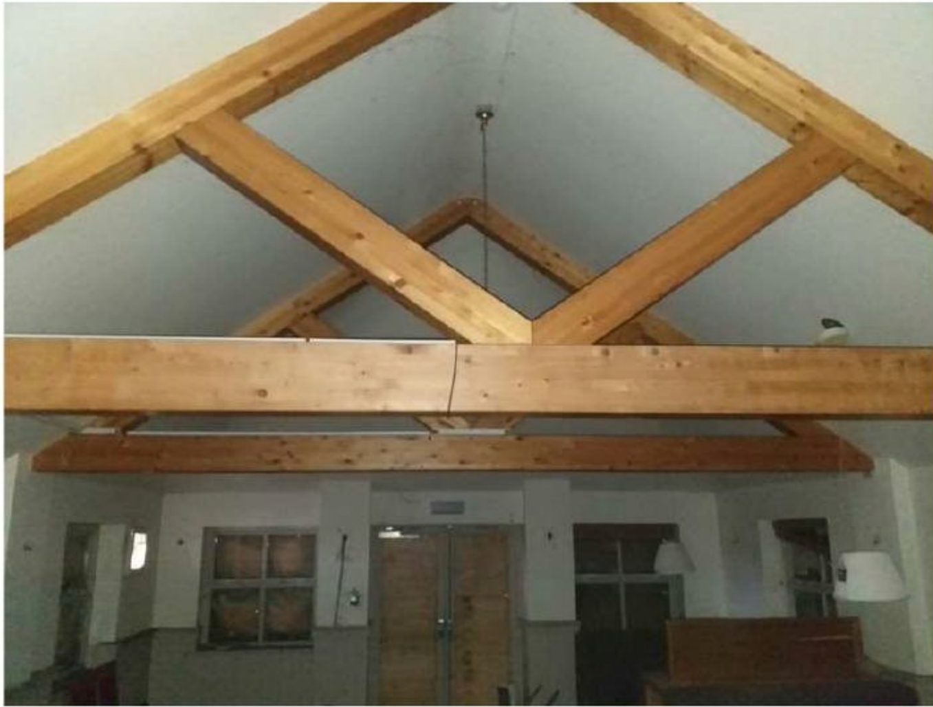
Vaulted ceiling in southern section of building
