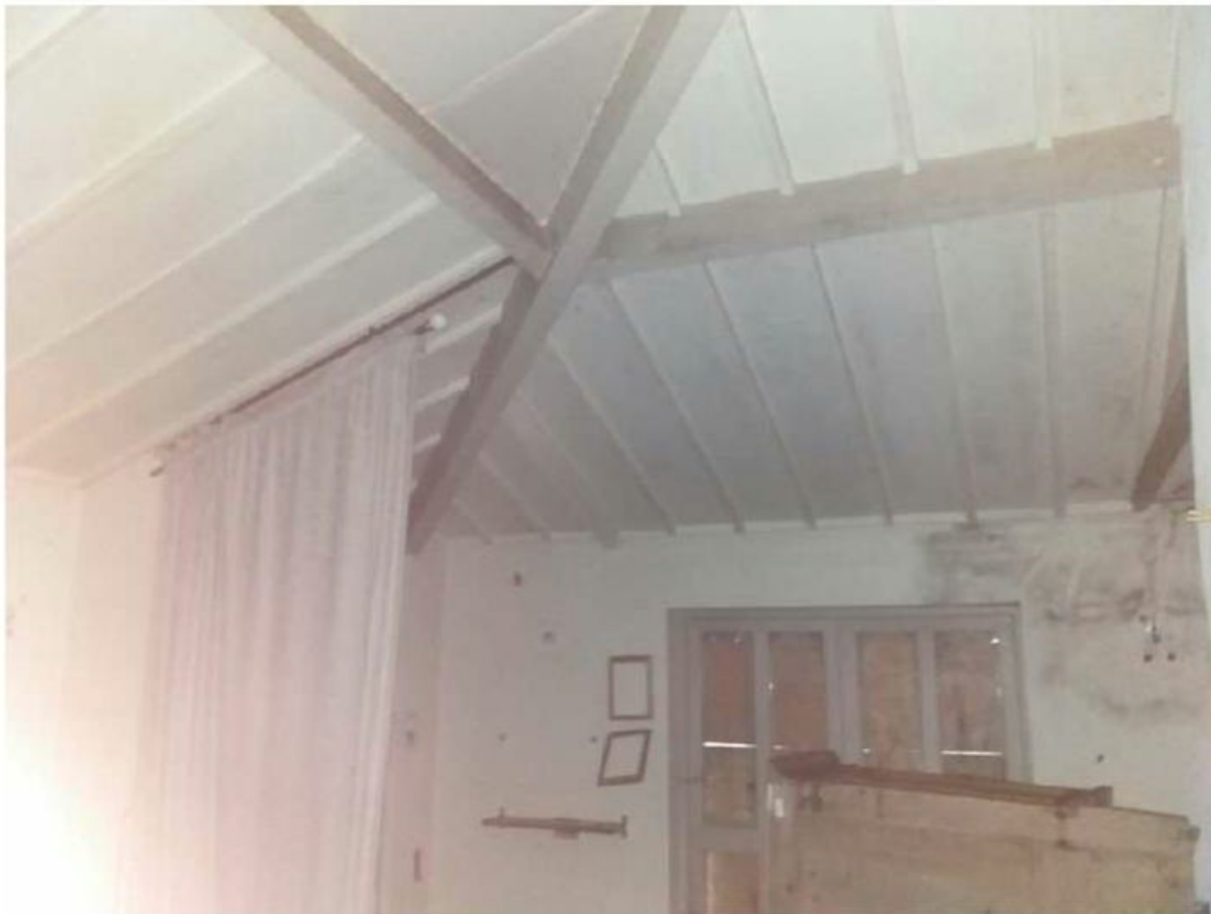
Vaulted ceiling in northern section of building
