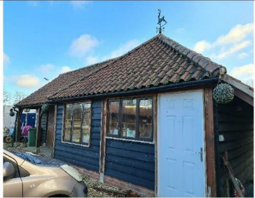
Structure 2. Office with windows on right and store room on left.
