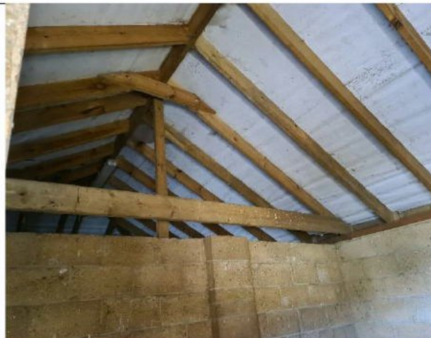
Structure 1- Internal of stable block with breathable roofing membrane visible under roof tiles. No void present
