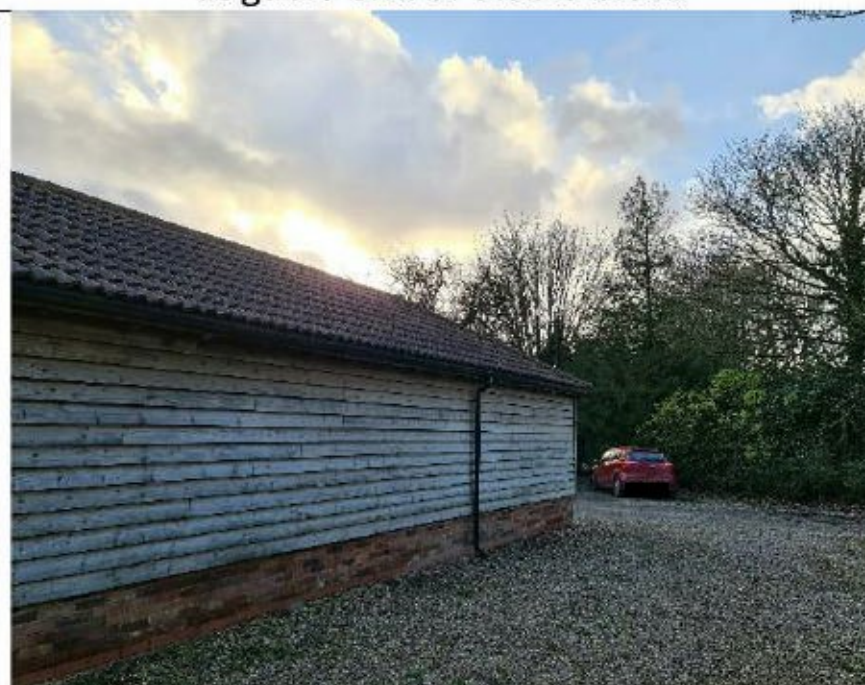
Structure 1- external timber cladding.
