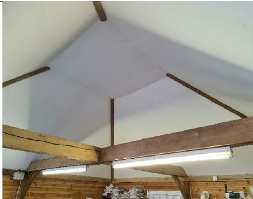
Structure 2- west side renovated office space.
