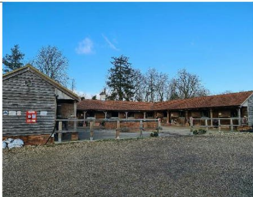
Structure 1- Stable block with timber clad walls and pantile roof. Hard standing present around stable block
