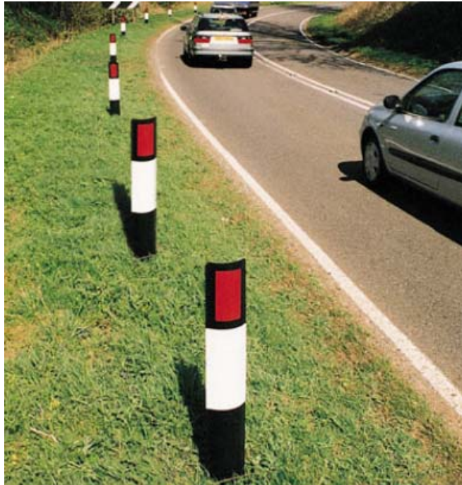
Insert 5.2: Example of flexible verge markers to prevent parking on the verge.
