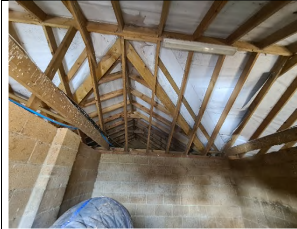
Structure 1- Roof structure where store room joins to stable block.
