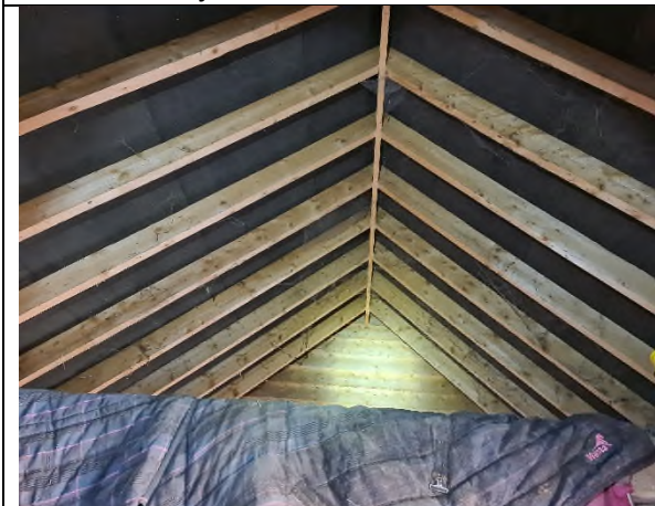
Structure 2- Eastern side internal, roof felt visible.
