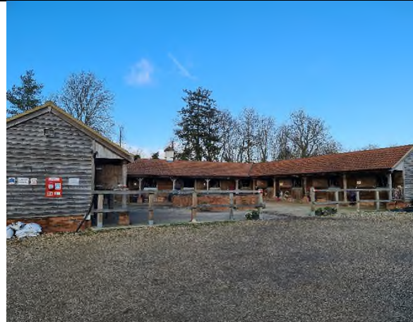
Structure 1- Stable block with timber clad walls and pantile roof. Hard standing present around stable block
