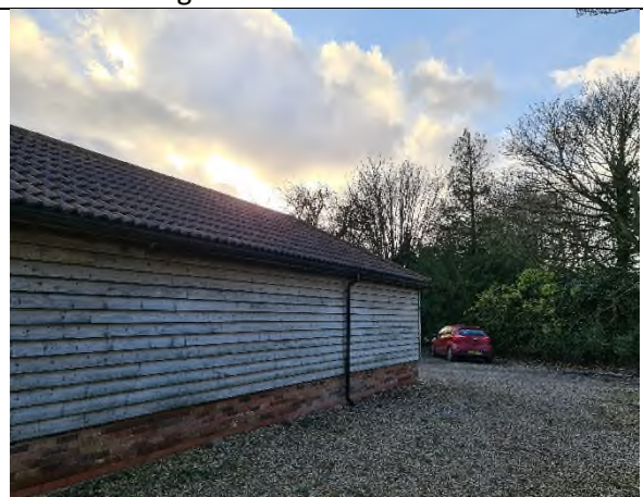
Structure 1- external timber cladding.
