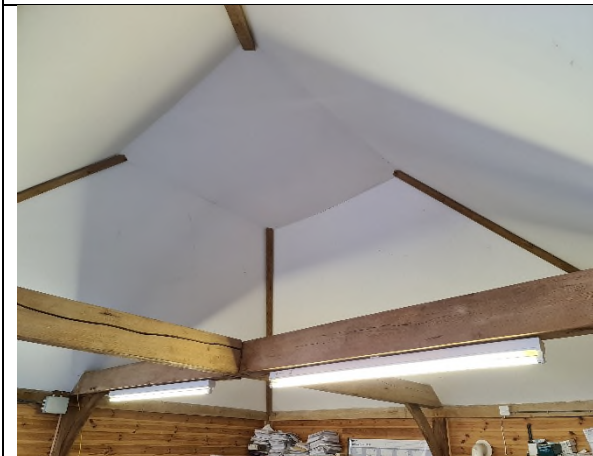
Structure 2- west side renovated office space.
