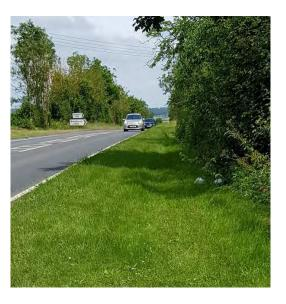
The A143, east of the development access, has a slight rolling vertical crest curve, with a raised verge area along the southern side of the A143. This may reduce the forward visibility (stopping sight distance) to and for pedestrians crossing at the bus stop hardstanding. Reduced forward visibility may lead to pedestrian to vehicle collisions, particularly as this section of the A143 is on a straight alignment and vehicle speeds appeared to be high.
