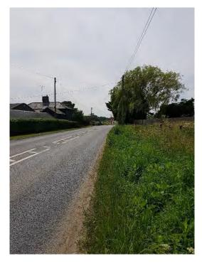
At the crossing, there is reduced forward visibility (stopping sight distance) to the east to / from the northern crossing point. Reduced forward visibility may lead to poor crossing decisions by users and to pedestrian / cyclist to vehicle collisions.
