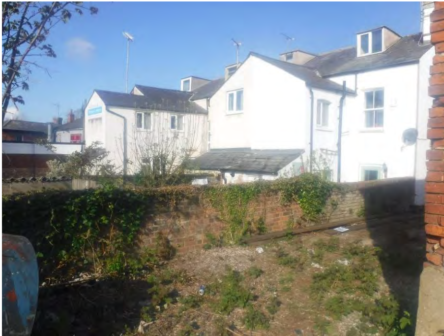
Photograph 20: View of adjacent properties to the southwest.
