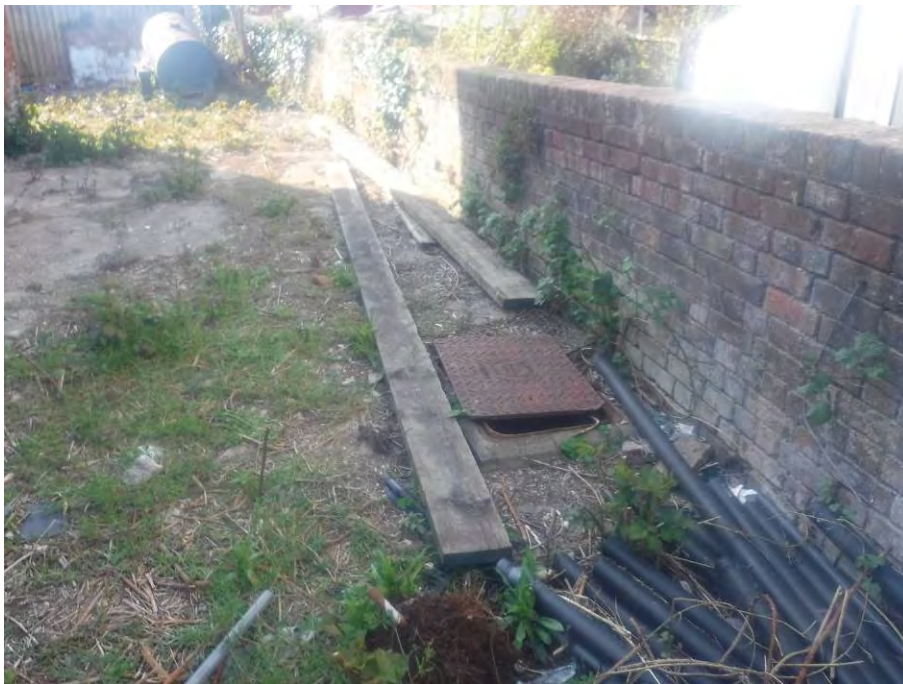
Photograph 8: General view, on-site drain cover and discarded pipe.
