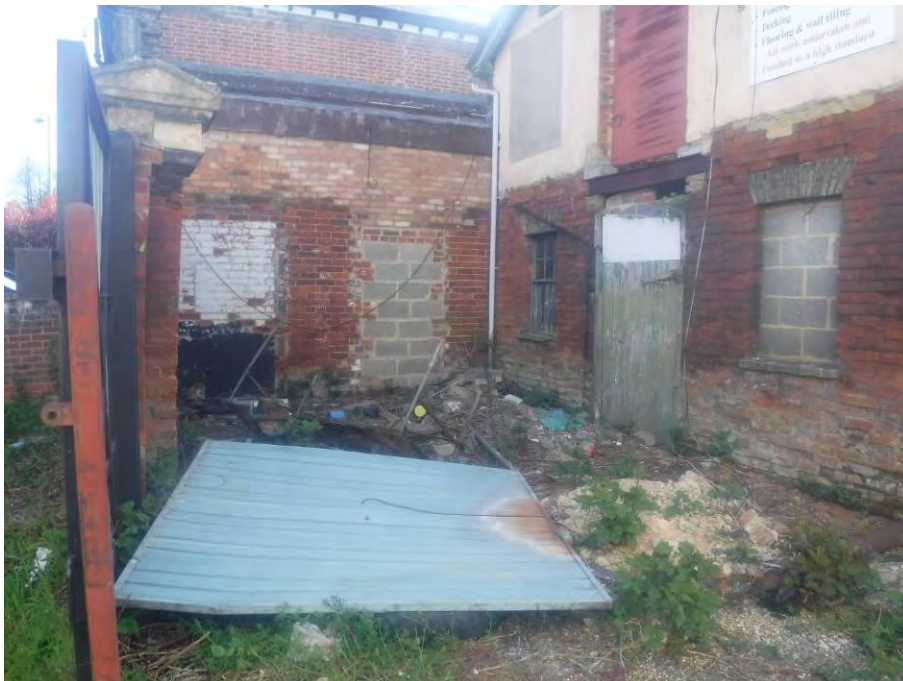
Photograph 12: General view of the front yard: garage door, old table, old engine (partially obscured by the upturned table).
