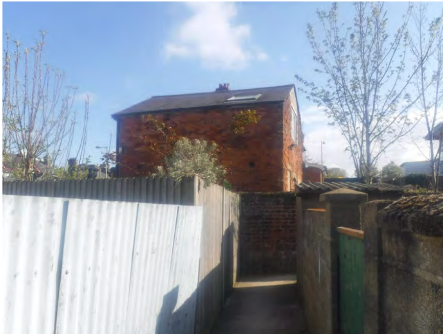
Photograph 5: The on-site building looking from the southwest.
