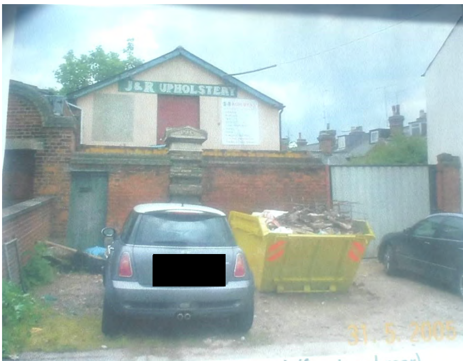
P3. Showing the frontage during the ownership of a land drilling contractor in 2005. (Image provided by Mr Ray Oakley and reproduced by permission).
