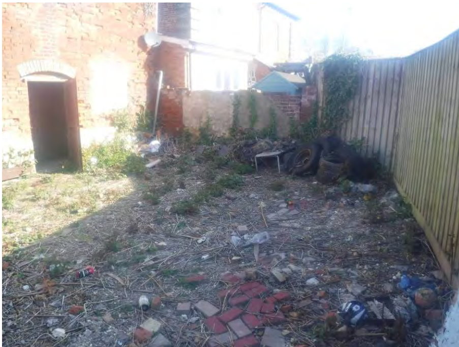
Photograph 18: General view of the rear yard.
