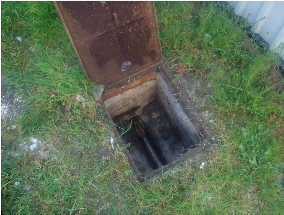
Photograph 9: On-site drain at the front of the site.
