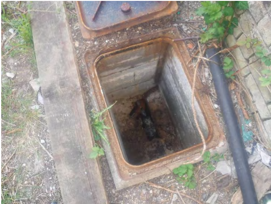
Photograph 10: On-site drain on the southwest side of the site.
