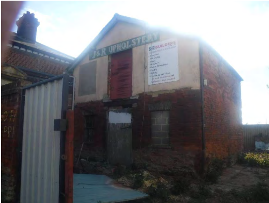
Photograph 11: General view of the existing building.
