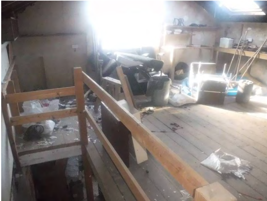
Photograph 27: General view inside the building on the first floor (1).
