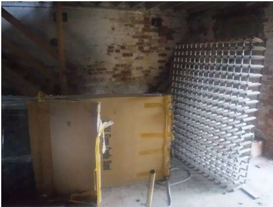
Photograph 25: General view inside the building on the ground floor (3).
