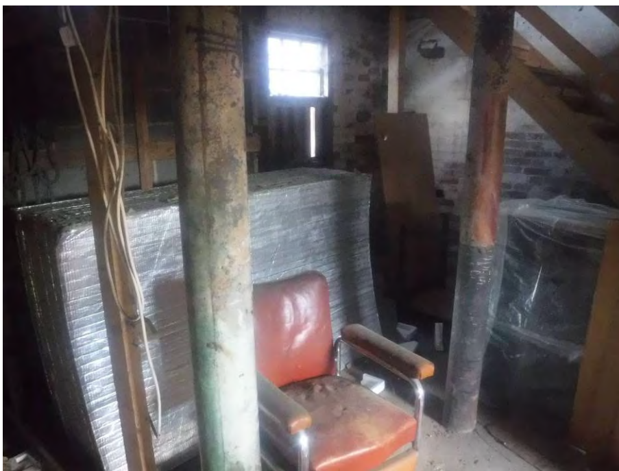
Photograph 26: General view inside the building on the ground floor (4).
