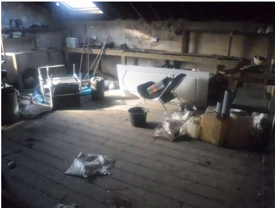
Photograph 28: General view inside the building on the first floor (2).
