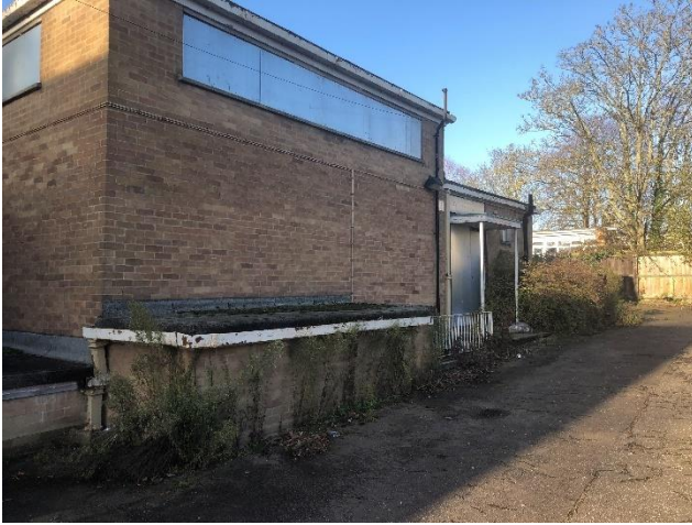
Photograph 3.3 Area of ephemeral/short perennial at the eastern side of building B2
