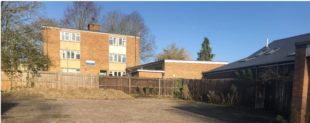
Photograph 3.2 Example of hardstanding found onsite.
