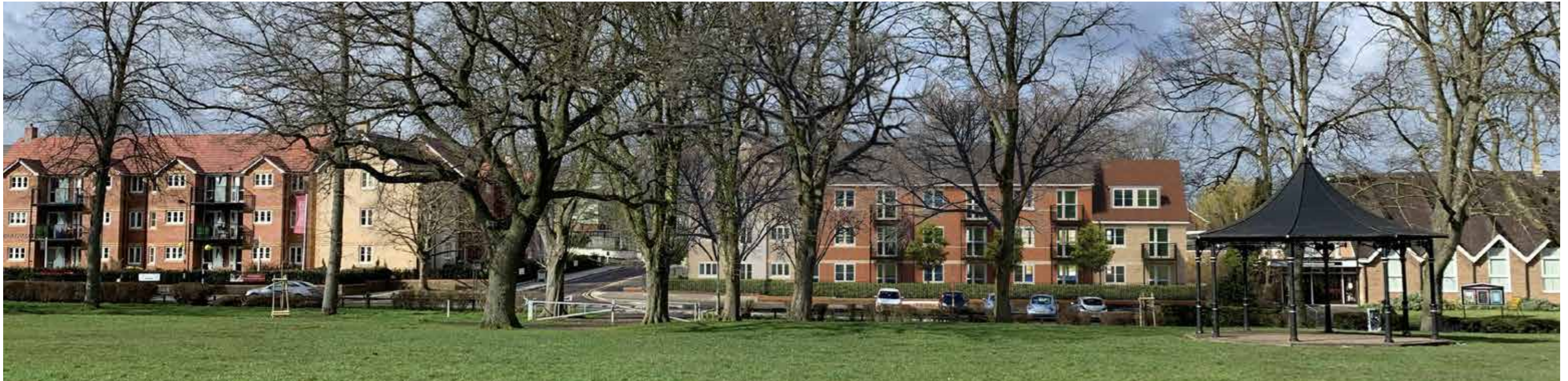
CGI of the proposed development viewed from Haverhill Recreation Ground. The development sits comfortably between Weaver's Lodge on the left and the Methodist Church to the right.
