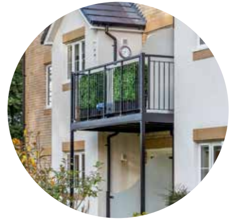
Brushed stainless steel balconies
