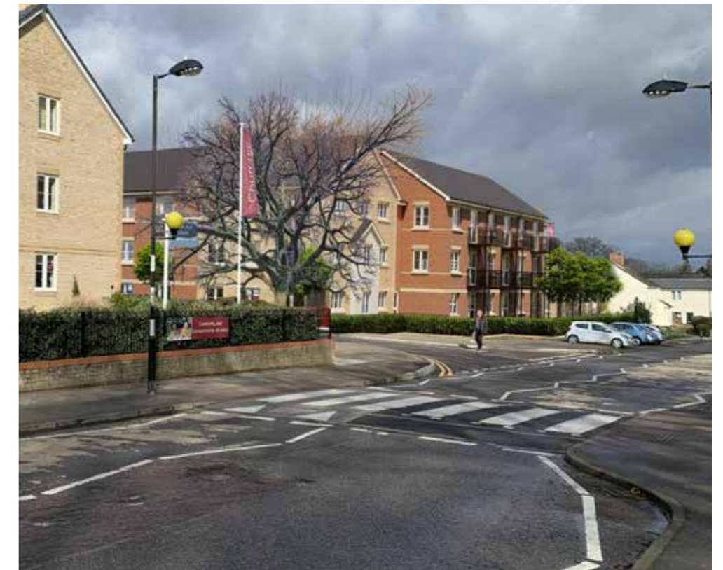
CGI of the proposed development viewed from the east of the site, looking down Camps Road
