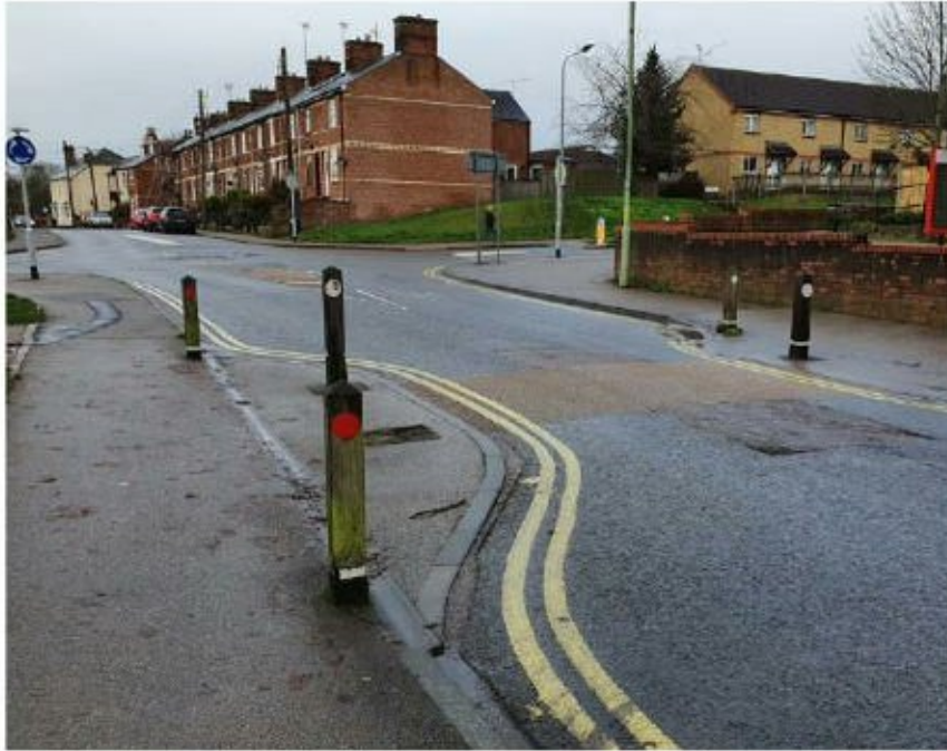
Photograph 7: Build outs on Camps Road 80m west of service road junction with Camps Road
