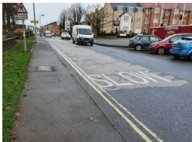
Photograph 10: Footway adjacent to southern side of Camps Road
