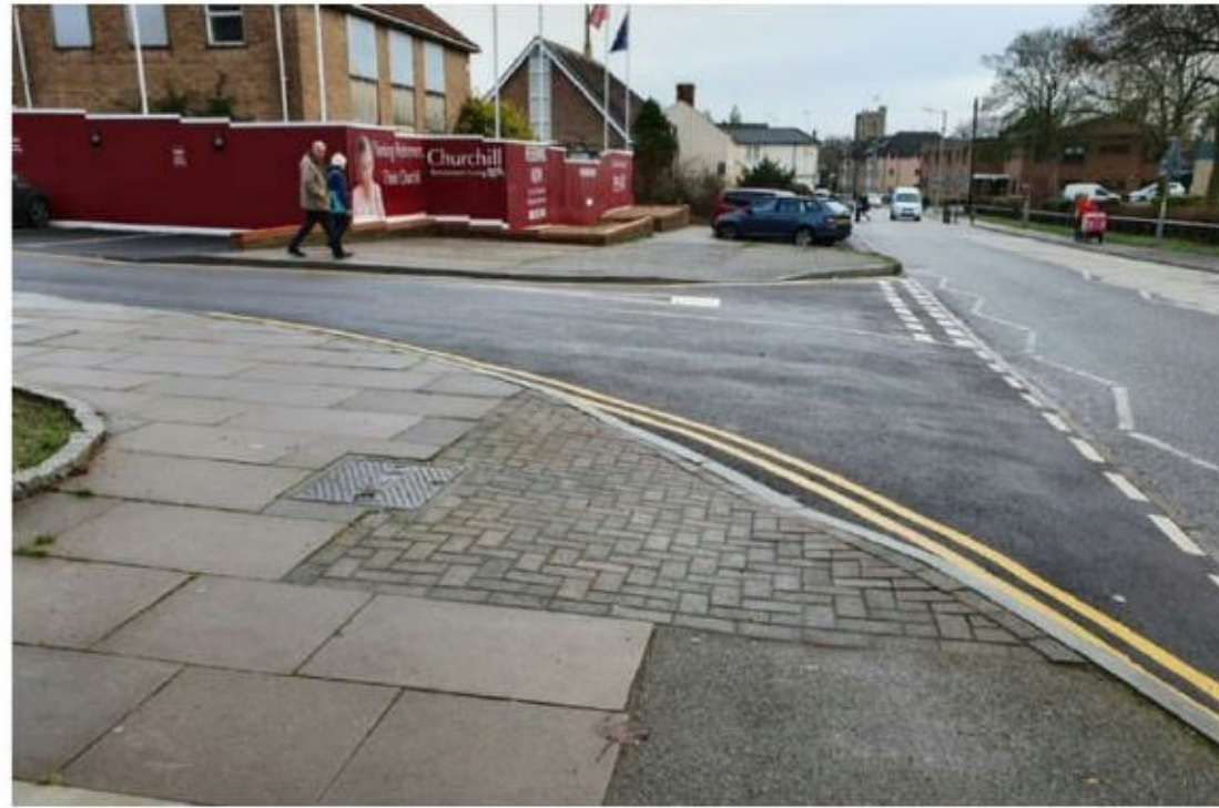
Photograph 11: Dropped kerb crossing on service access junction with Camps Road
