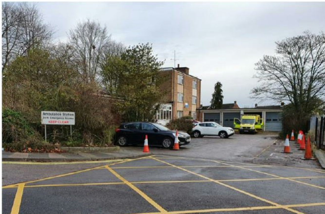
Photograph 3: Ambulance station access adjacent to northern site access onto service road
