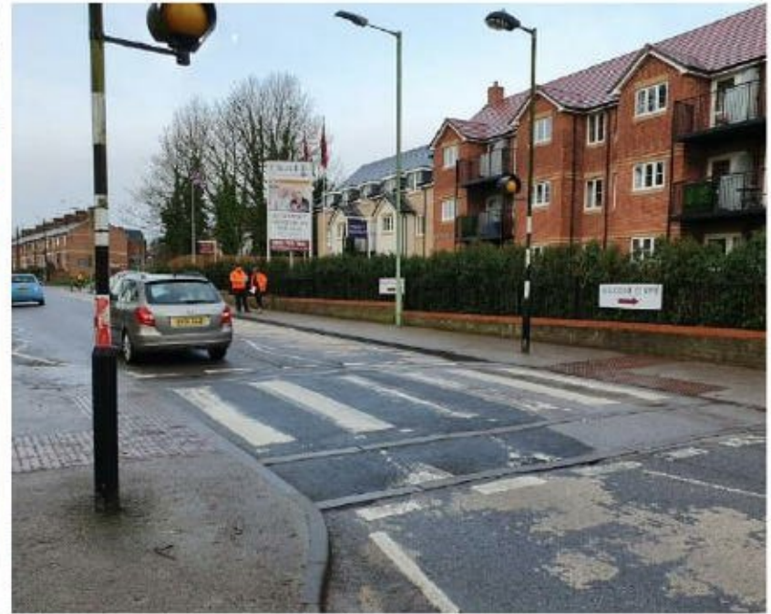
Photograph 8: Raised zebra crossing 15m west of service road junction with Camps Road
