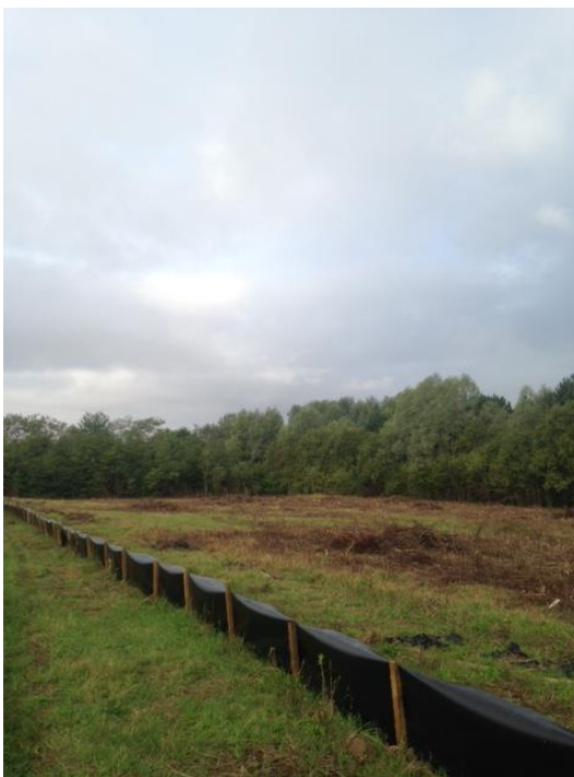
Photograph 3 – Receptor site and new fence line
