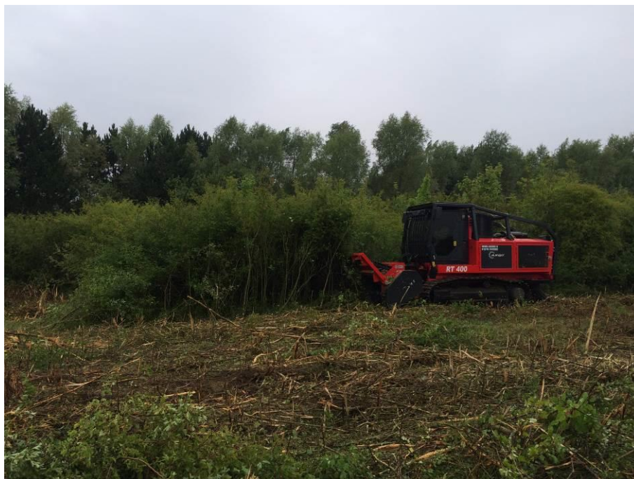
Photograph 1 – Management works occurring in the receptor site
