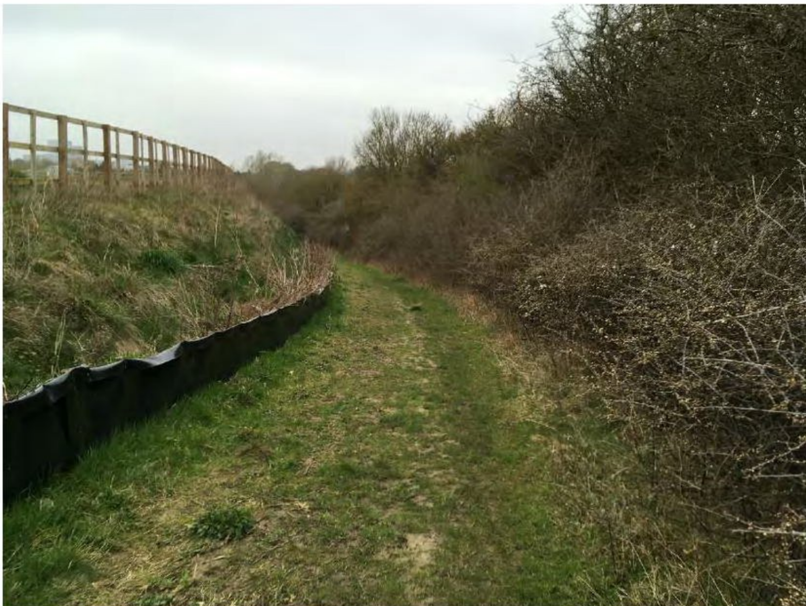
Photograph 4 – Reptile exclusion fencing adjacent to the north of the Site
