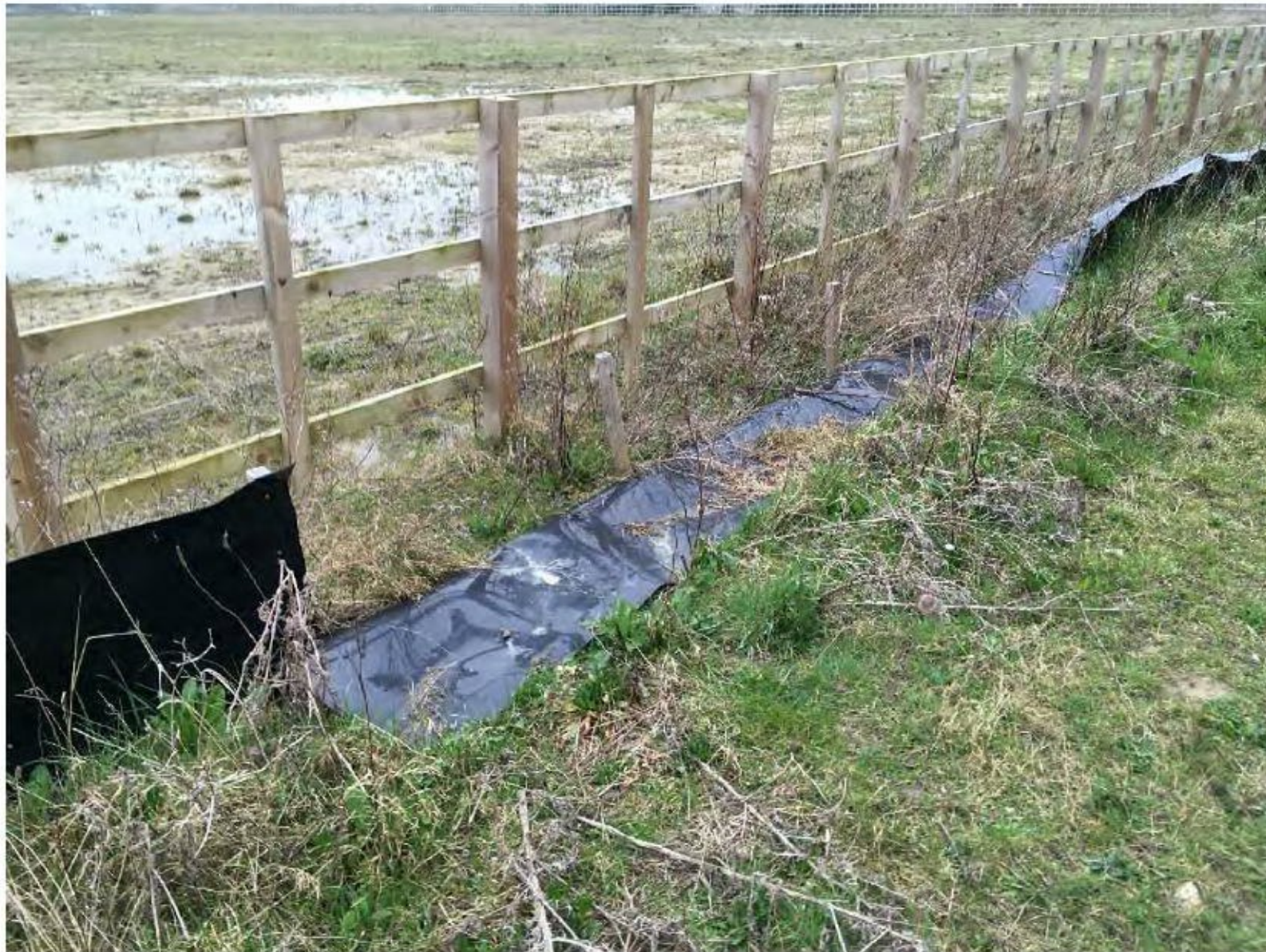
Photograph 5 – Example of damage to reptile fencing
