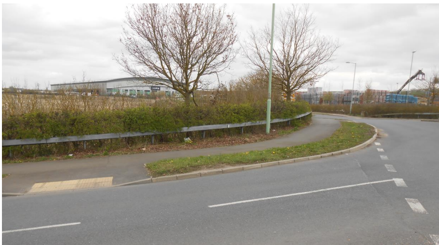
C View West back along Icen Way towards Haverhill Business Park
