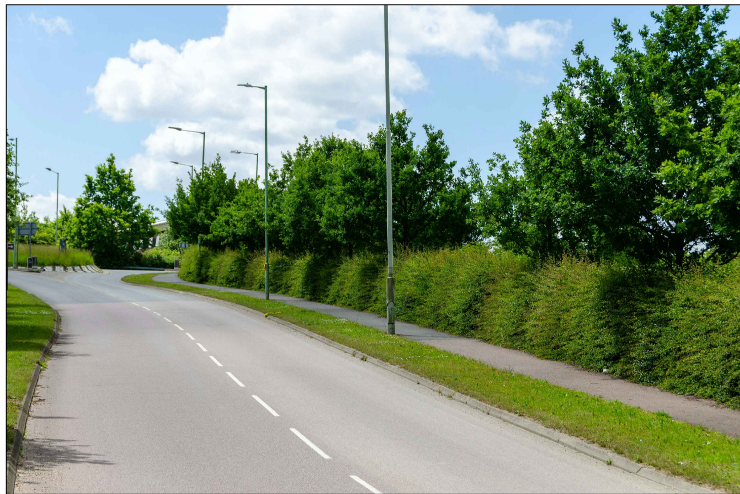
VIEW 01 - FROM BUMPSTEAD ROAD LOOKING SOUTH WEST AS EXISTING
