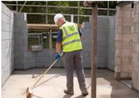
1) Clear debris from work area.
