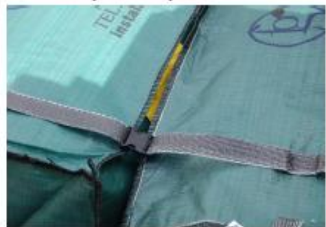
4) Ensure bags are secured tightly together
