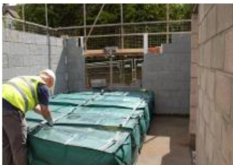
5) Continue to assemble until the floor area is covered.
