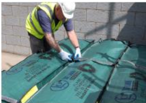
3) Check clips are free of debris
