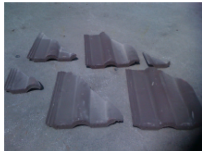
Off-cuts to be re-used on hips
