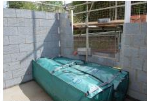
2) Load bags into work area and place in position.
