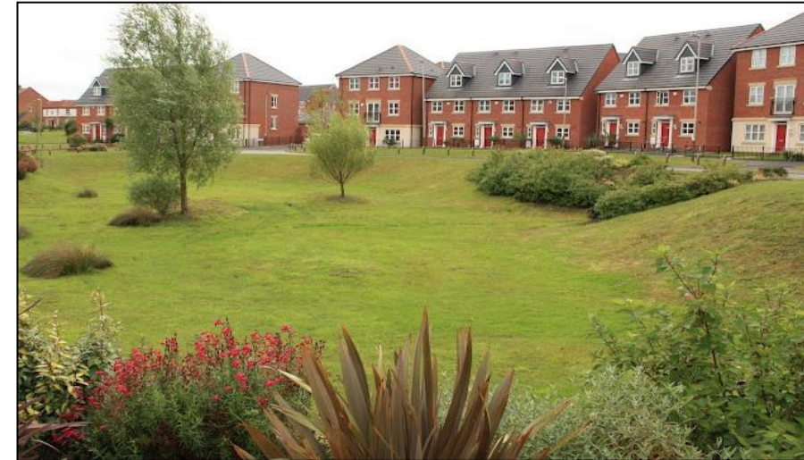
Figure 39: Example of a dry SUDS basin
