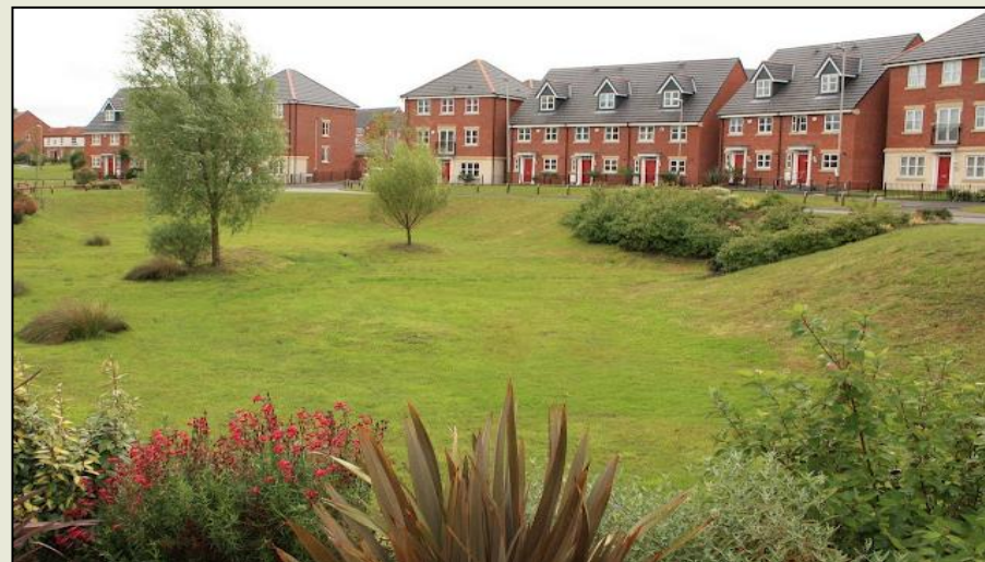
Figure 12: Example of an accessible SUDs basin
