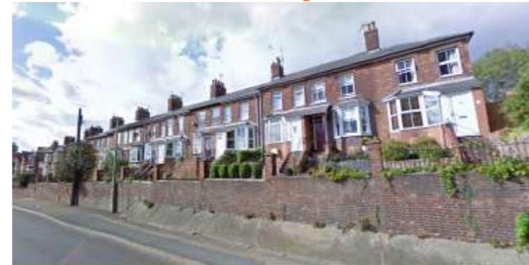
Photo 1: Victorian Terraced Housing
