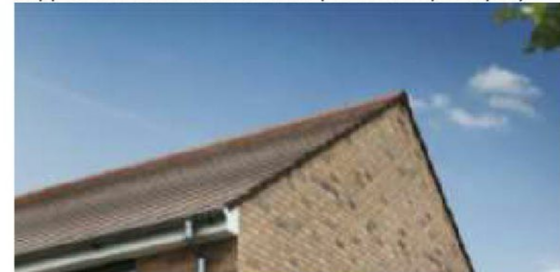
Clipped eaves for clean and simple contemporary style
