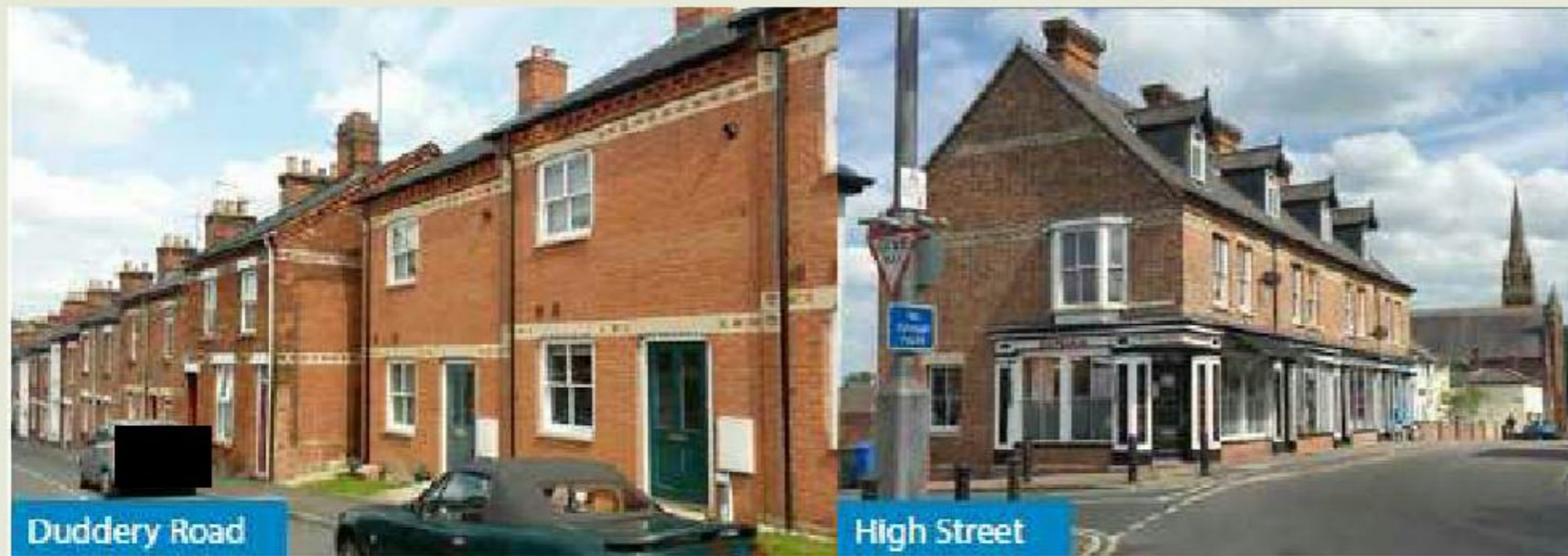
Examples of polychromatic brick detailing
