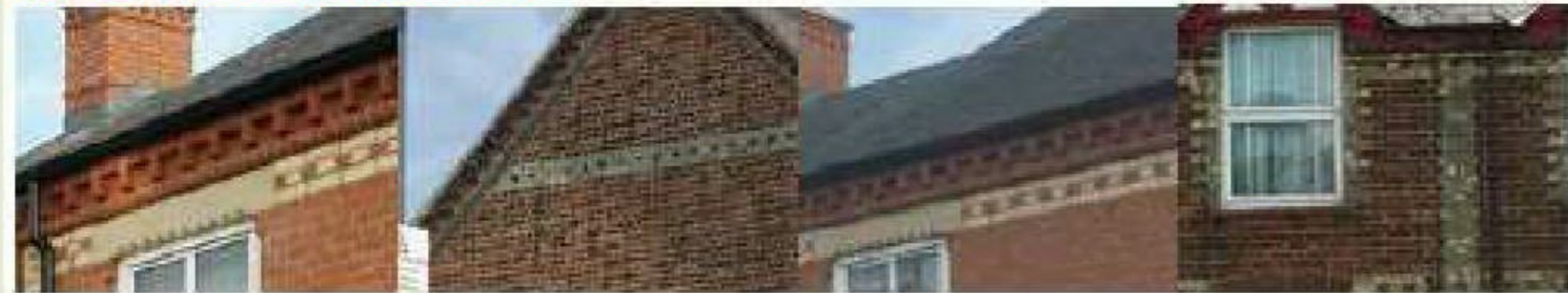
Examples of polychromatic brick detailing
