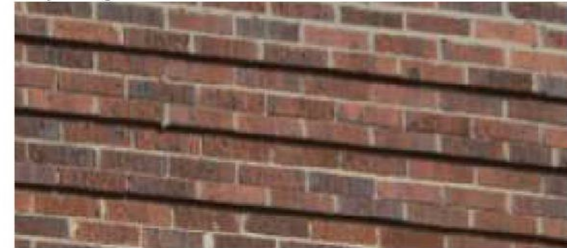
Projecting Brick Band Detail
