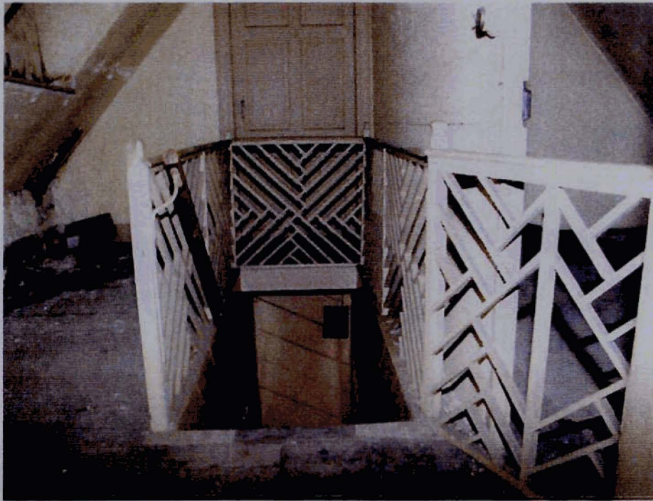
Plate 5 Attic staircase and gate in Building 1 taken from E
