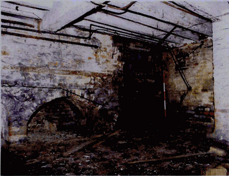
Plate 2 Eastern bay of basement in Building 1 taken from SW
