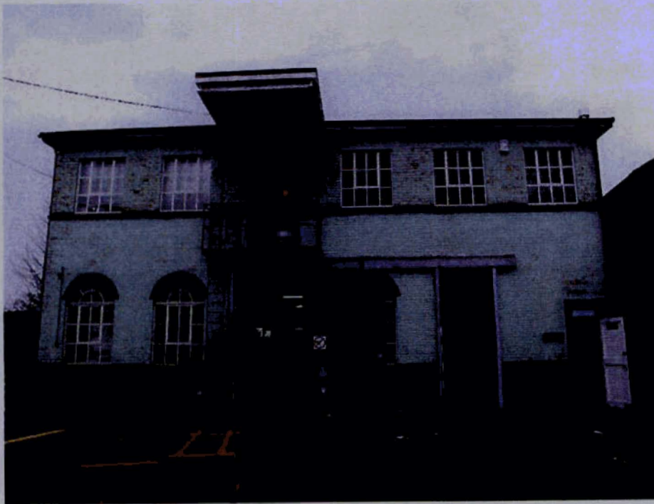
Plate 15 Exterior west elevation of Building 5 taken for W
