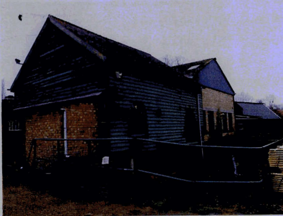
Plate 16 Exterior east and north elevation of Building 6 taken from NE
