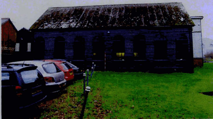
Plate 14 Exterior south elevation of Building 4 taken from S
