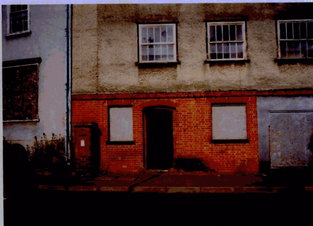
15. Detail of front elevation to Silk Mill adjacent to Hamlet House.
