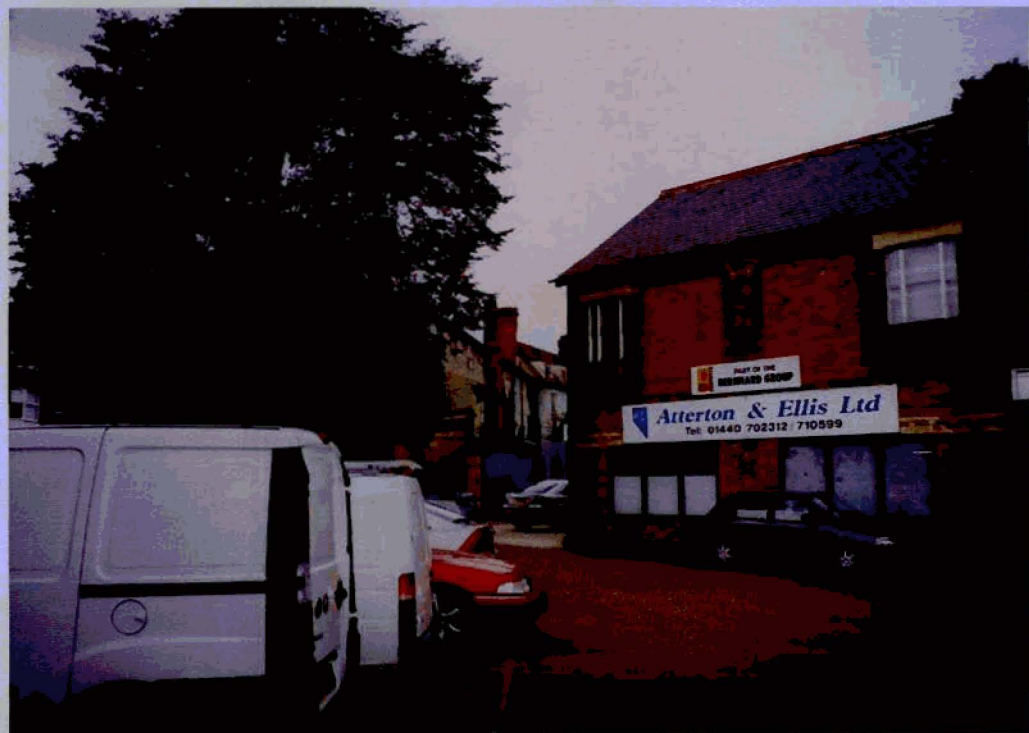
20. Detail of original office building showing historic alterations to façade.
