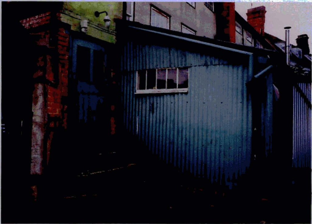
17. Rear façade of Silk Mill – extensions to be removed and Mill converted.
