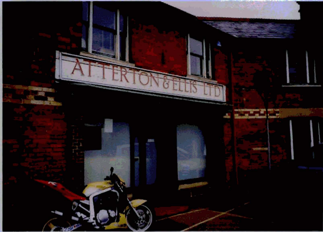
19. Detail of original shop front to Victorian building. Extended within and now functioning as workshop.
