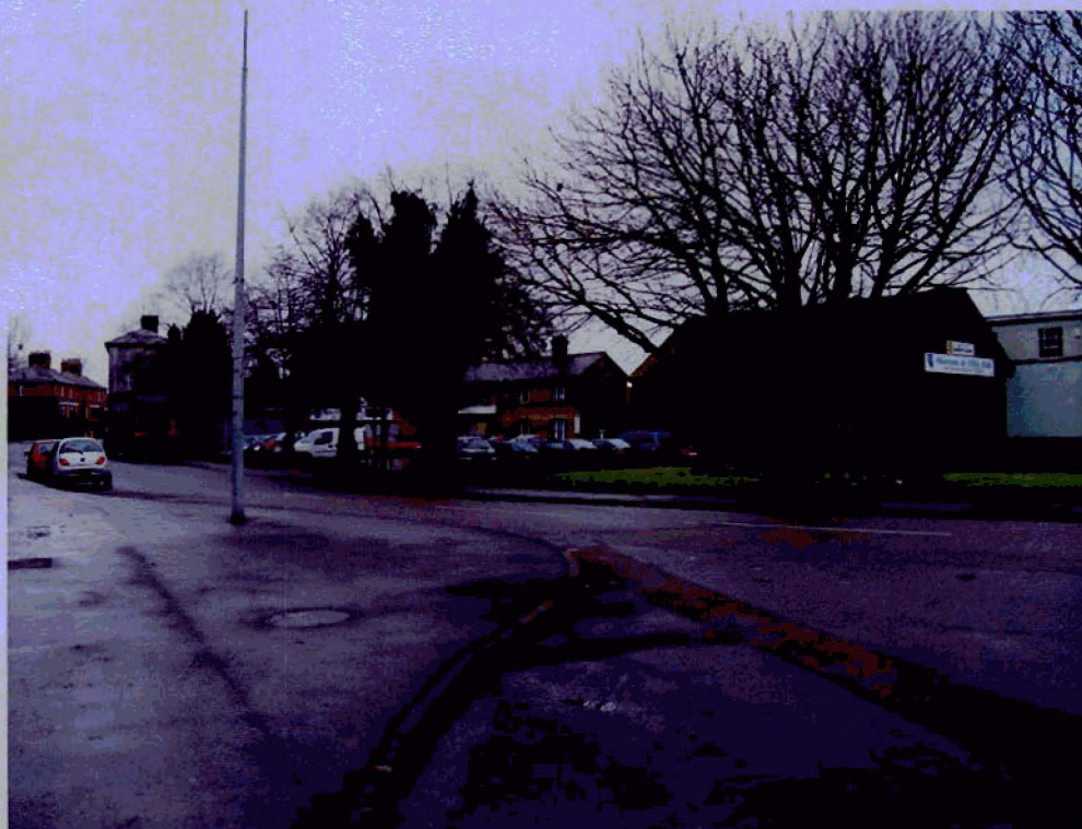
6. Looking West showing main building line to Hamlet Road and relationship between Silk Mill, existing offices and timber clad building
