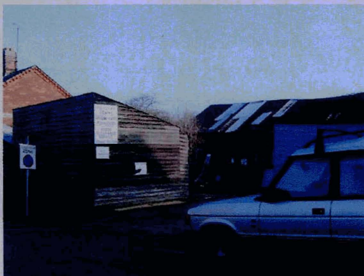
Run down industrial yard
