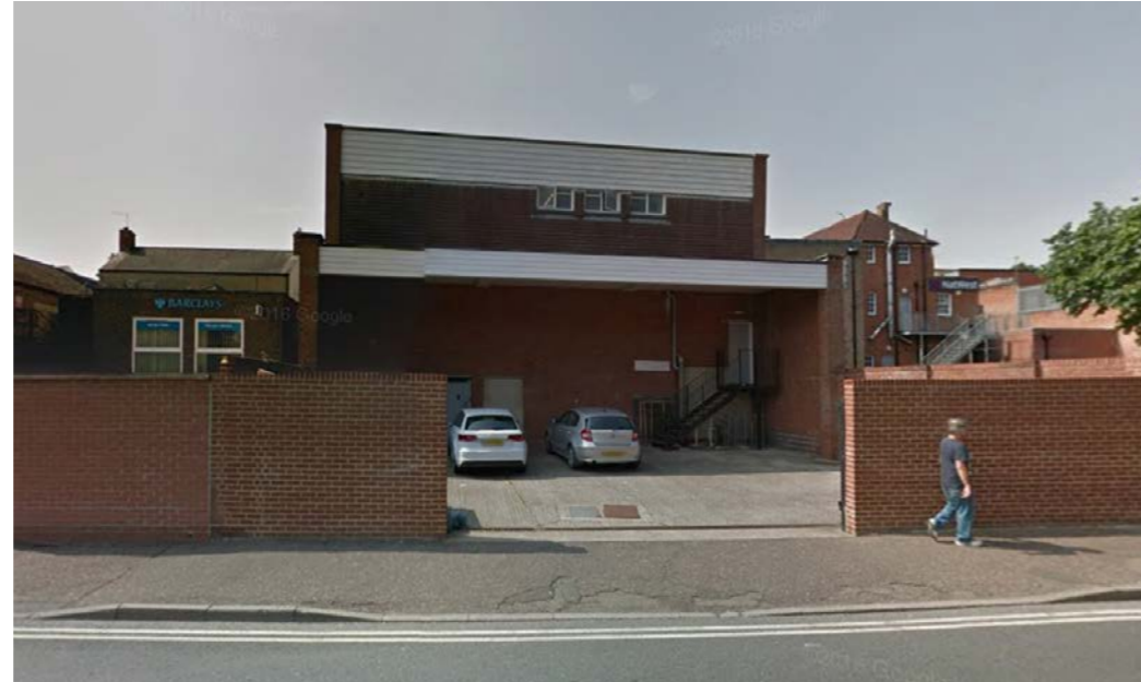
Brook Service Road Brick building with flat roof. Rear access for Dorothy Parking, Burton and Gavin's fast food.
