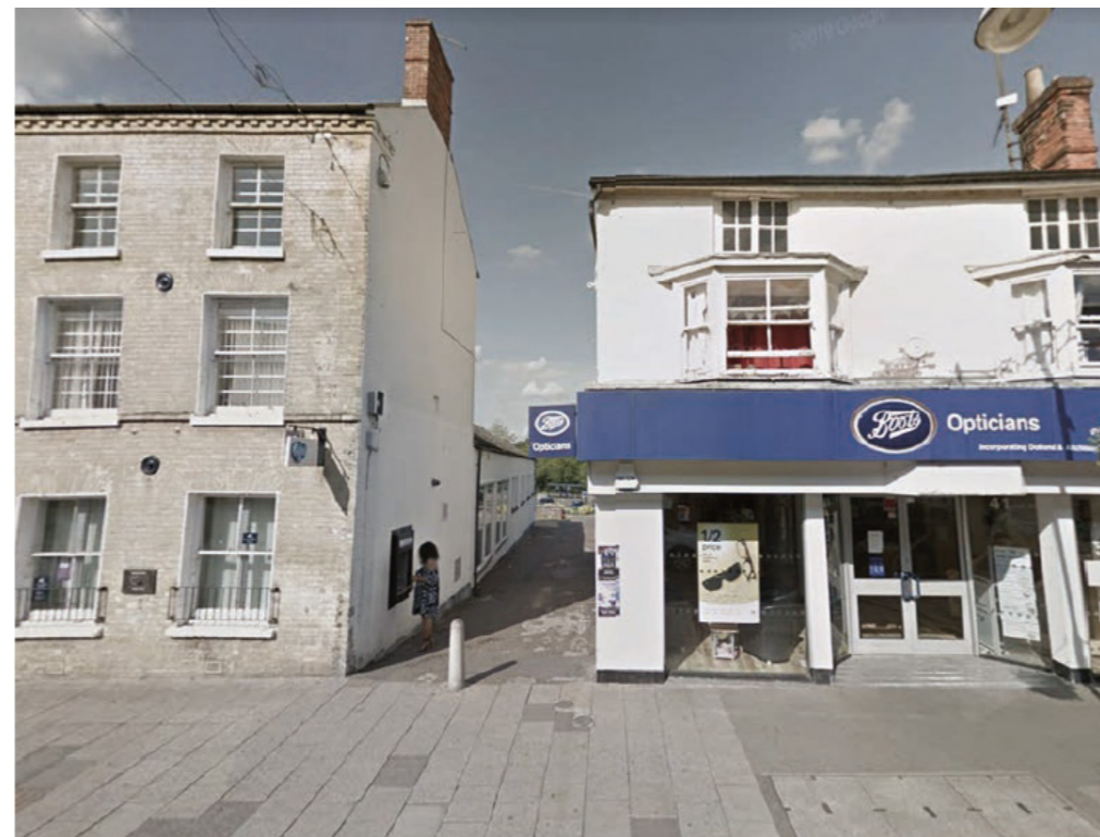
High Street Photograph - Pedestrian Access
