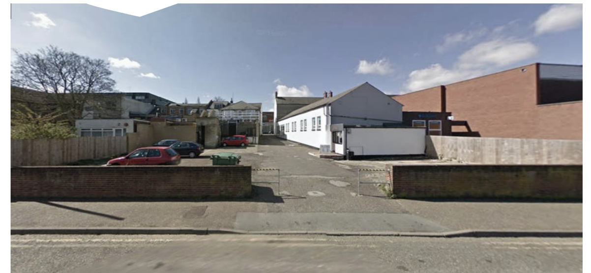
Barclays Bank - Rear access - Brook Service St Grad II listed building
