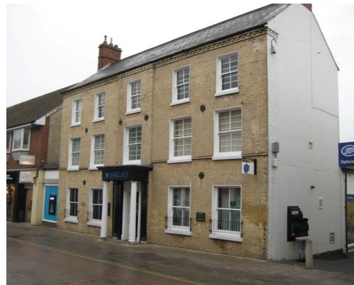
Barclays Bank- Front access- Market Hill Grad II listed building
