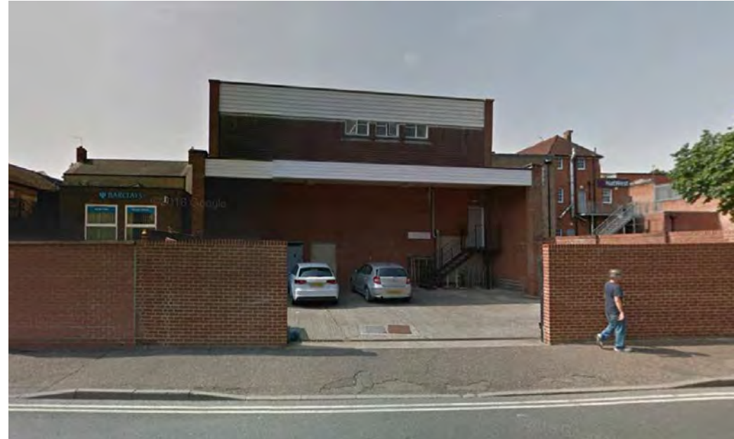
Brook Service Road Brick building with flat roof. Rear access for Dorothy Parking, Burton and Gavin's fast food.
