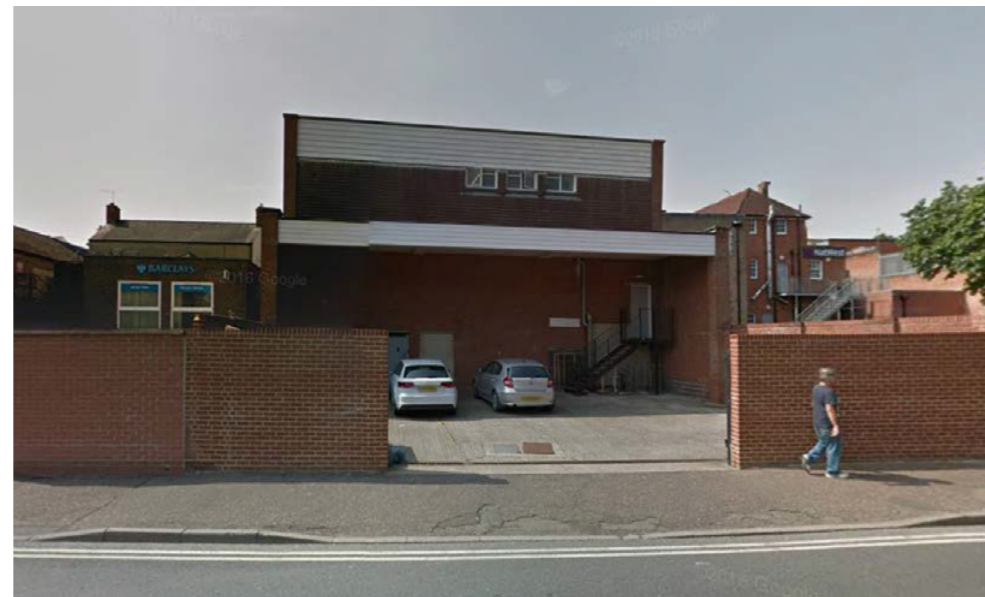
Brick building with flat roof. Rear access for Dorothy Parking, Burton and Gavin's fast food.
