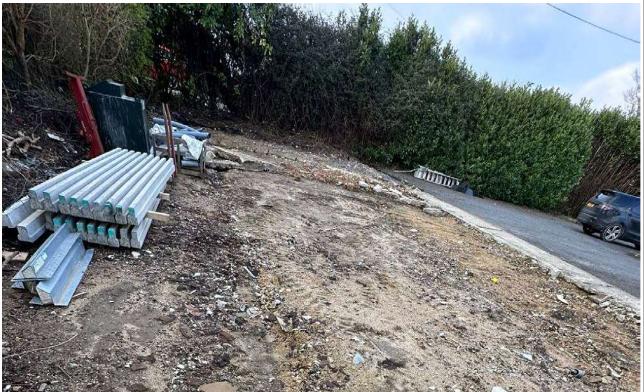
Photo 6: Construction materials stored in the south of the Site.
