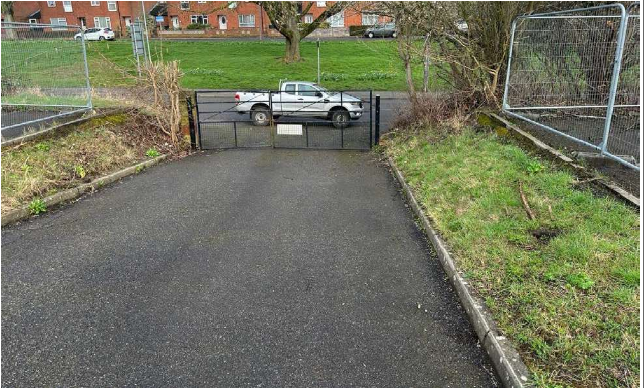
Photo 1: Site access from sloping driveway, with lockable gates at the base of the ramp.
