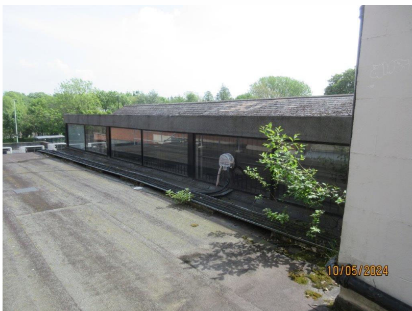
Photo 3: North light windows on flat roof
