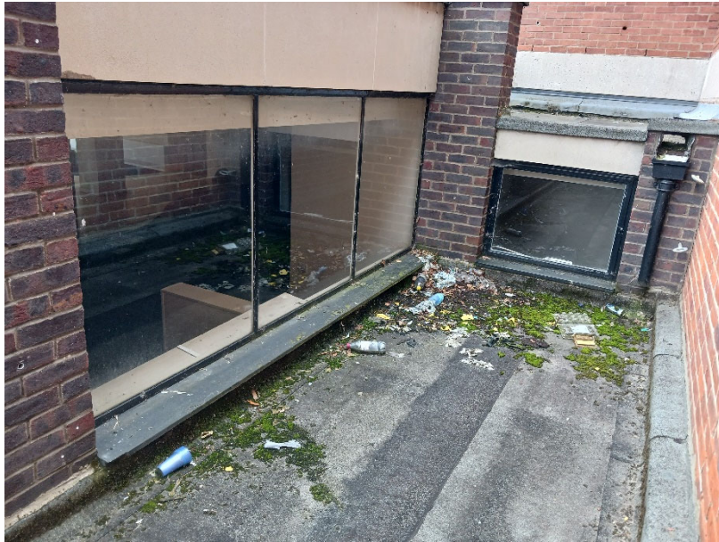
Photo 4: Windows to rear on lower flat roof
