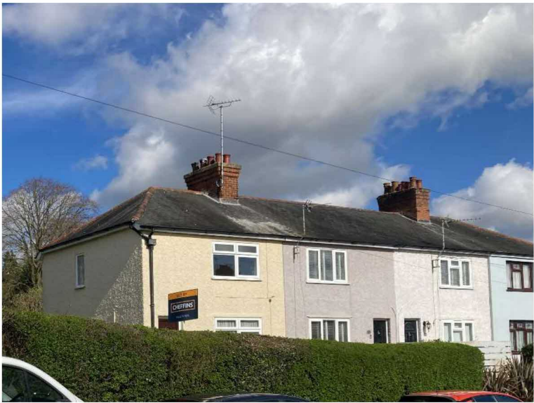
Existing end terrace house
