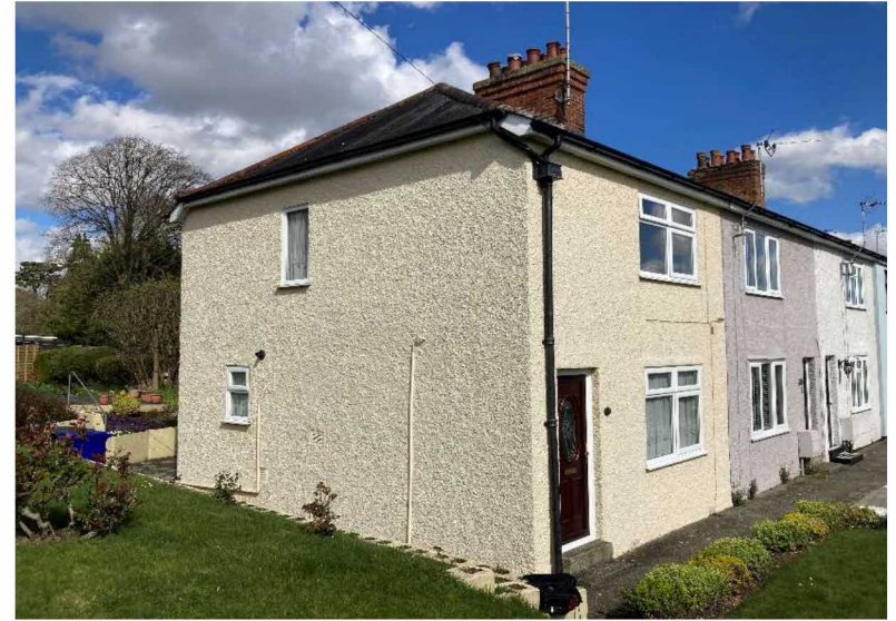
The Existing corner
