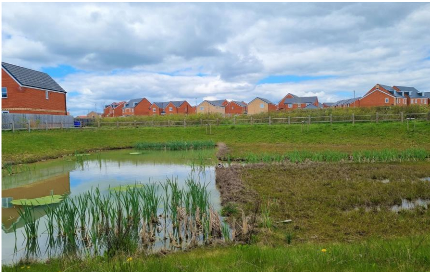
Figure 34: Basin within Phase 1 of the Haverhill Scheme.
