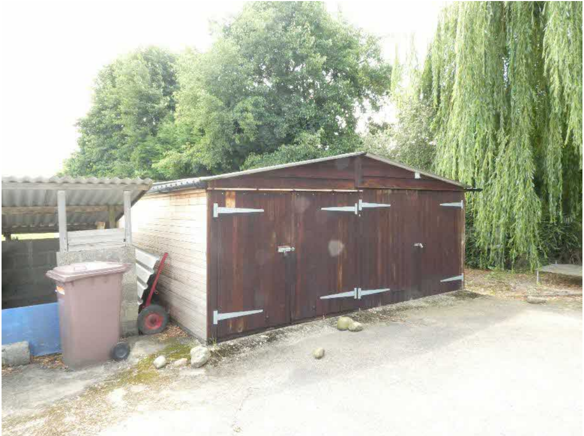
Photo 7, north and west aspects of building one, looking southeast.
