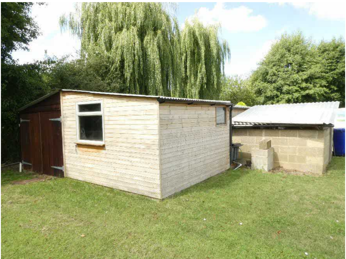
Photo 8, north and east aspects of building one, looking southeast.
