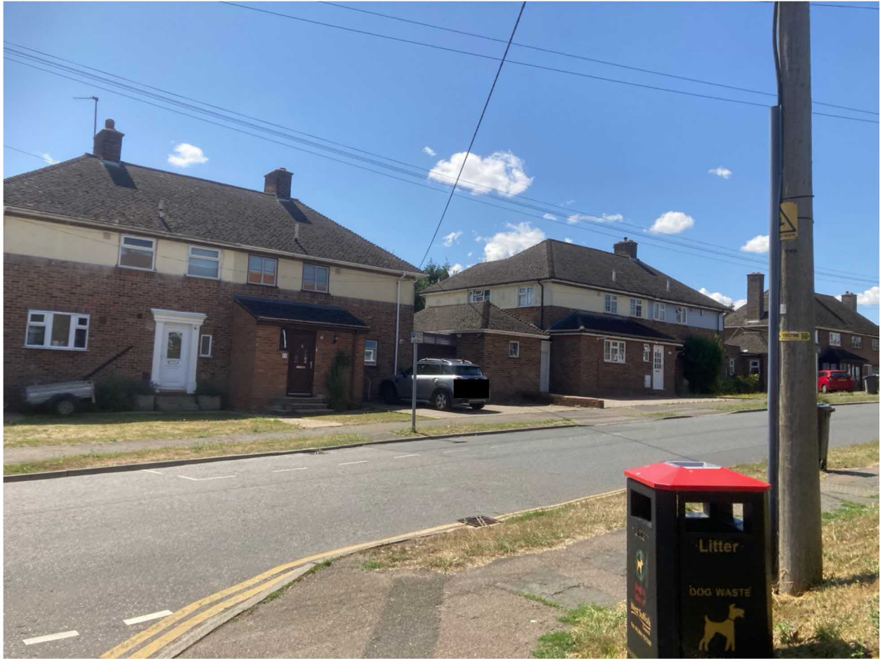
Above: Other examples of single storey front extensions within the area of Mill Hill with a combination of both hipped and mono-pitched roofs with concrete tiles and matching brickwork (as can be seen above).
