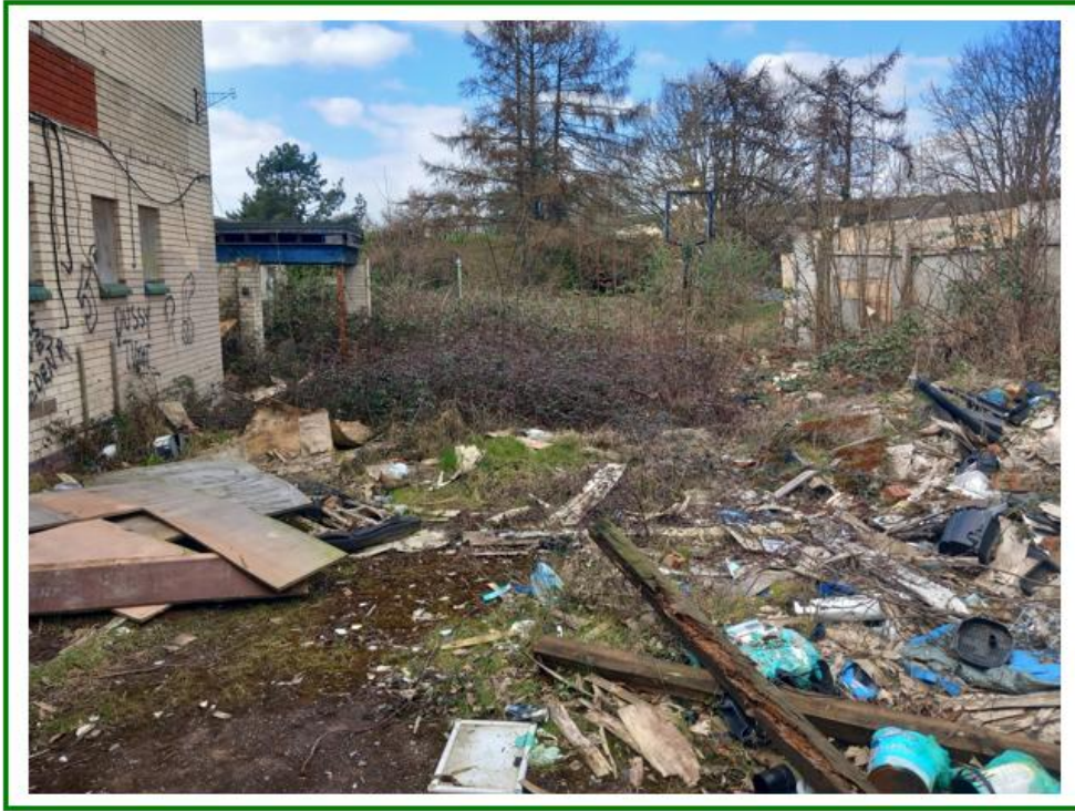
Photo No.10: Facing NW inside the hoarding and within the site boundary showing debris occupying NE extent of site
