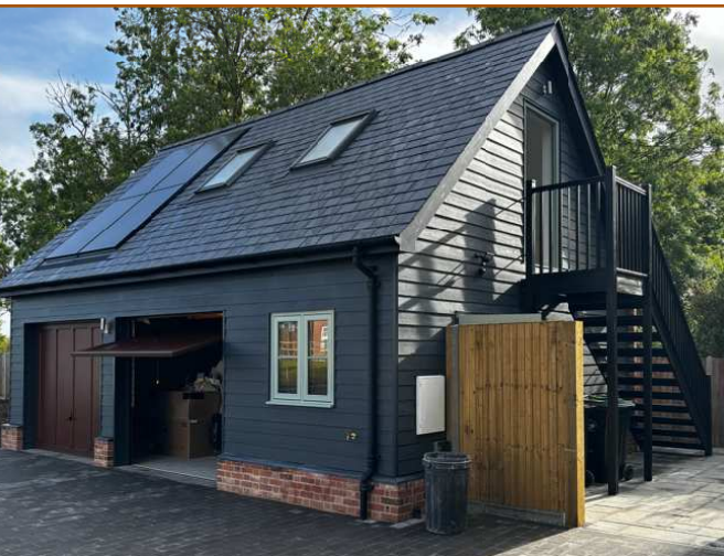
1. Example of Hardiplank Boarding to cartlodge building
